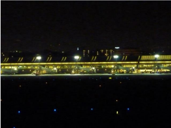
Figure 3.5-6: AIRPORT POLE LIGHTING – VIEW INSIDE AIRPORT CONTROL TO-ER - AT NIGHT
