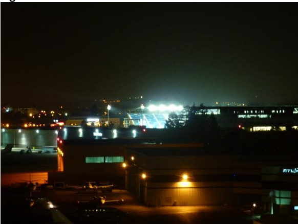
Figure 3.5-12: WAREHOUSE FLOOD LIGHTING – VIEW OUTSIDE AIRPORT CONTROL TOWER - AT NIGHT
