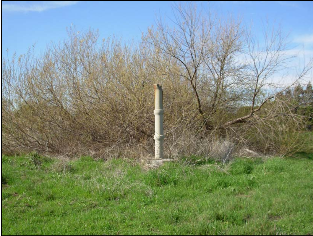
Photo 4: View of old water pipe on-site.
