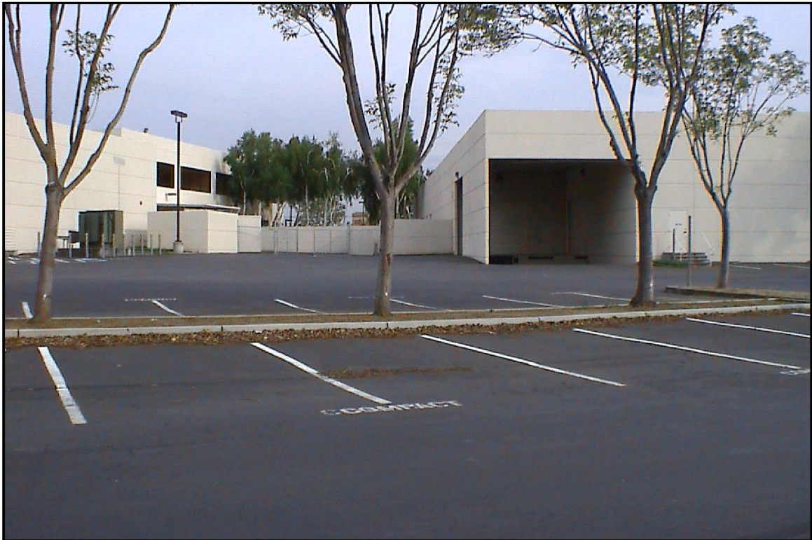
Photograph 2: View of project site from the northern boundary.
