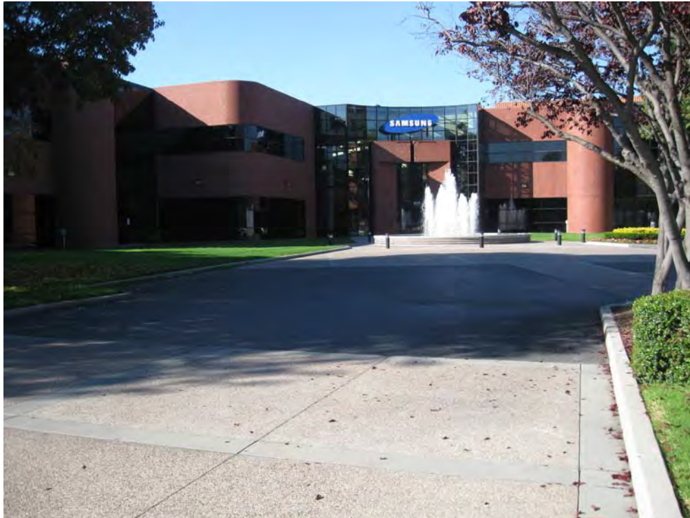
View of on-site building at 3655 North First Street
