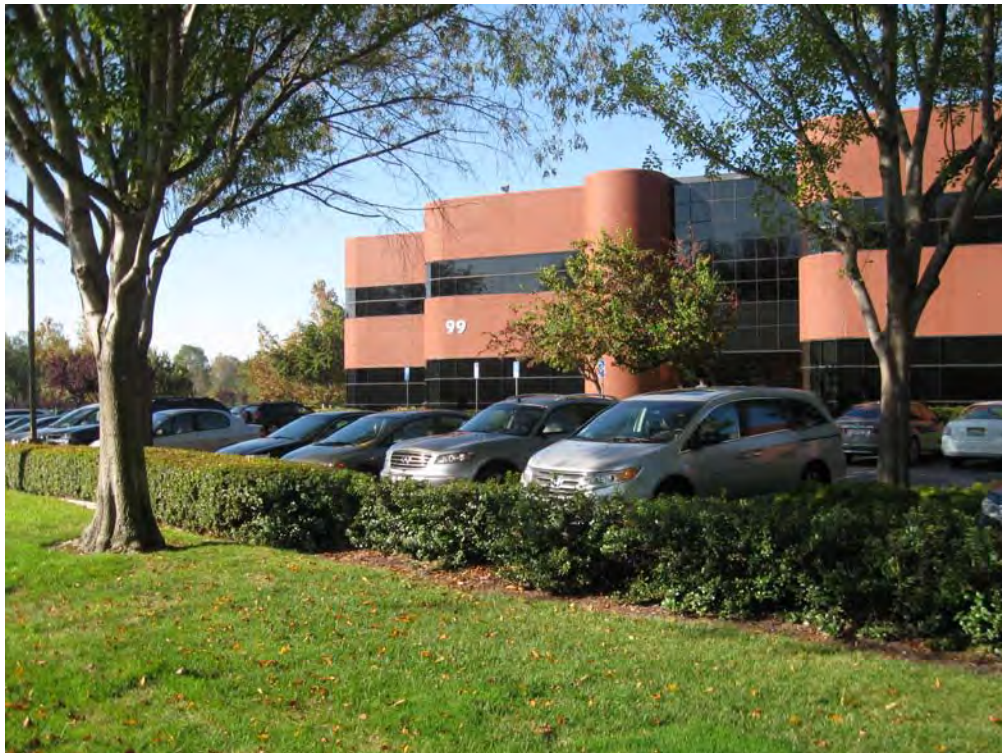
View of on-site building at 99 West Tasman Drive
