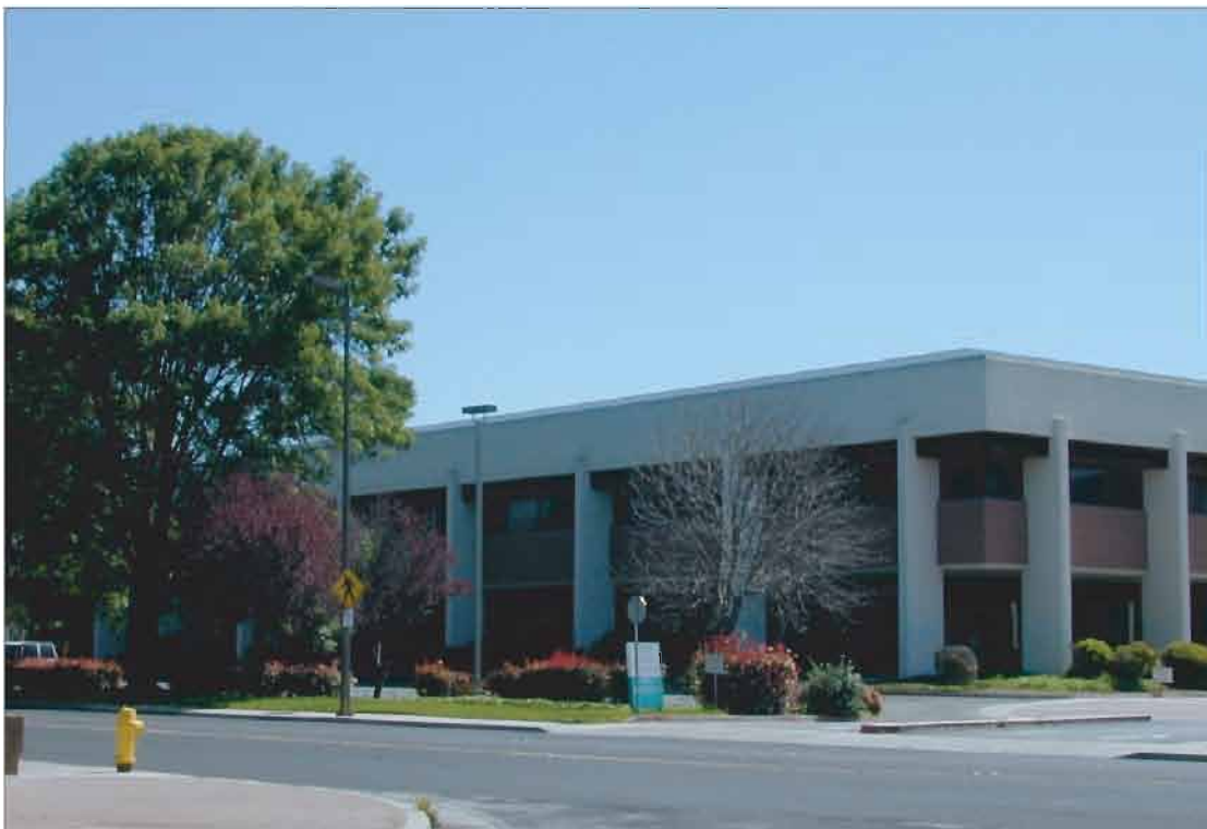
Photo 4 - View of Vista Montañã and Area 2 from the intersection of Renaissance Drive and Vista Montañã looking northeast.
