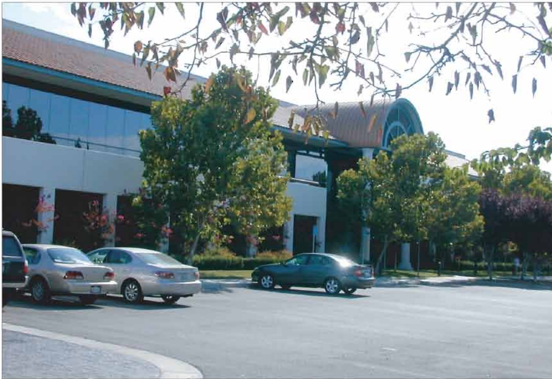
Photo 7 - View of Area 4 from the intersection of North First Street and Headquarters Drive looking southeast.
