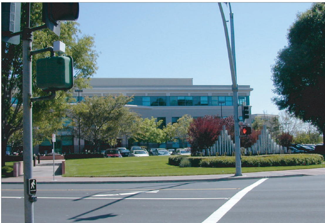
Photo 10 - View of office use located on the east side of Vista Montana, to the east of Area 3.
