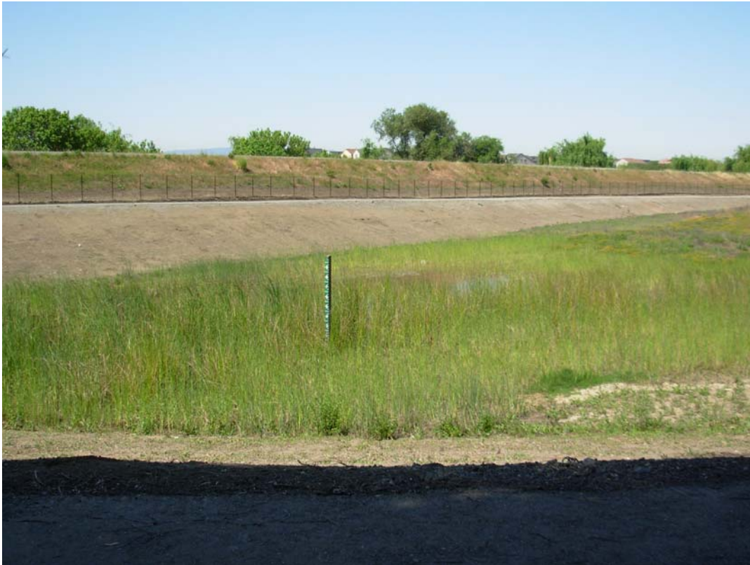
Photo 7 – View of detention basin located southwest of the site looking southwest.
