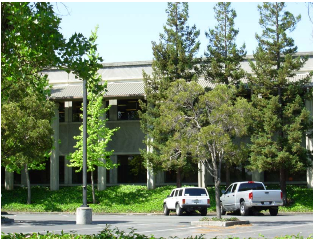
Photo 2 – View of project site from North First Street looking southwest.
