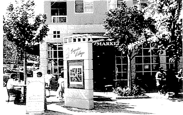
An active plaza is encouraged at the future West San Carlos LRT Station.
