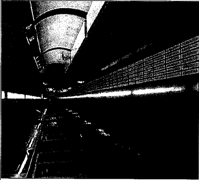
Pressurized emergency access stairs and tunnel ventilation shaft
