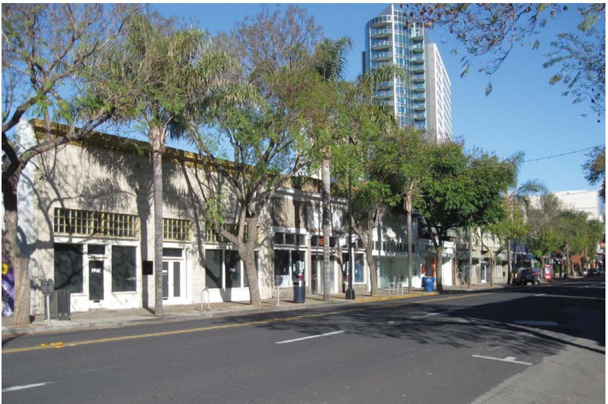
PHOTO 4: View of commercial buildings on the west side of S. First Street from the northeast corner of William and S. First Streets.
