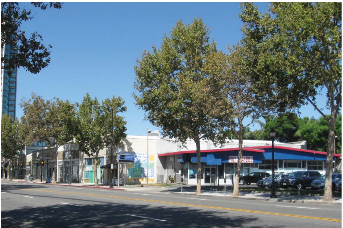
PHOTO 2: View of the project site looking northeast from the northwest corner of William and Market Streets.
