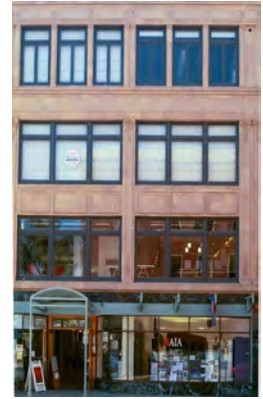
Fig 3-20 The Dohrman Building on First Street.
