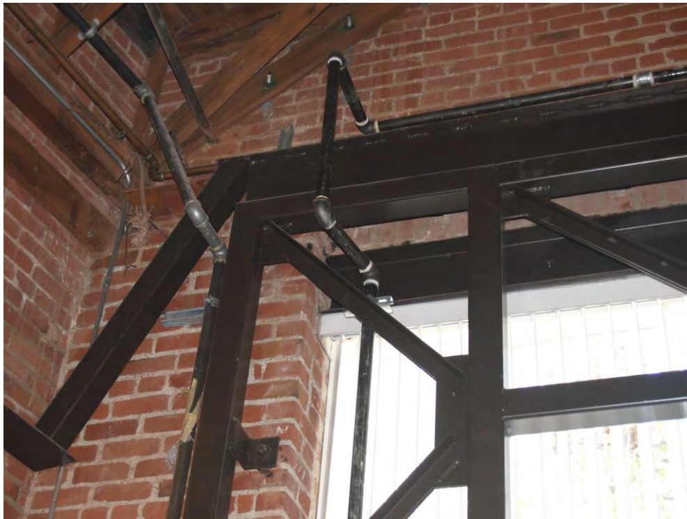
Internal structural reinforcement at façade.
