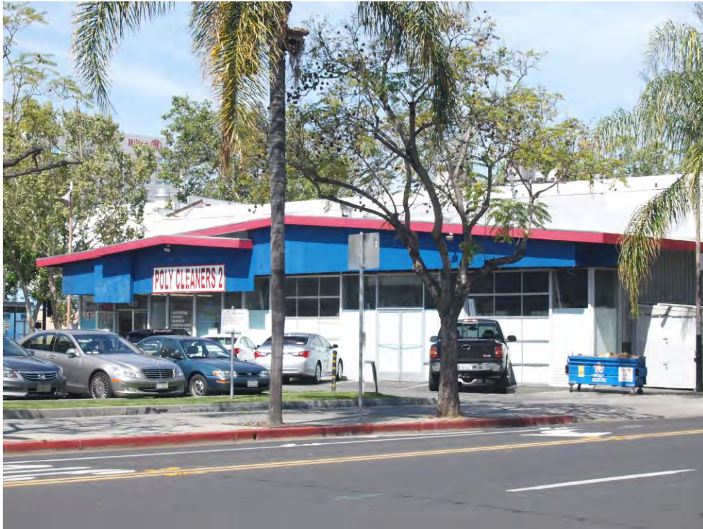
Main front elevation from South First Street, viewed facing northwest.
