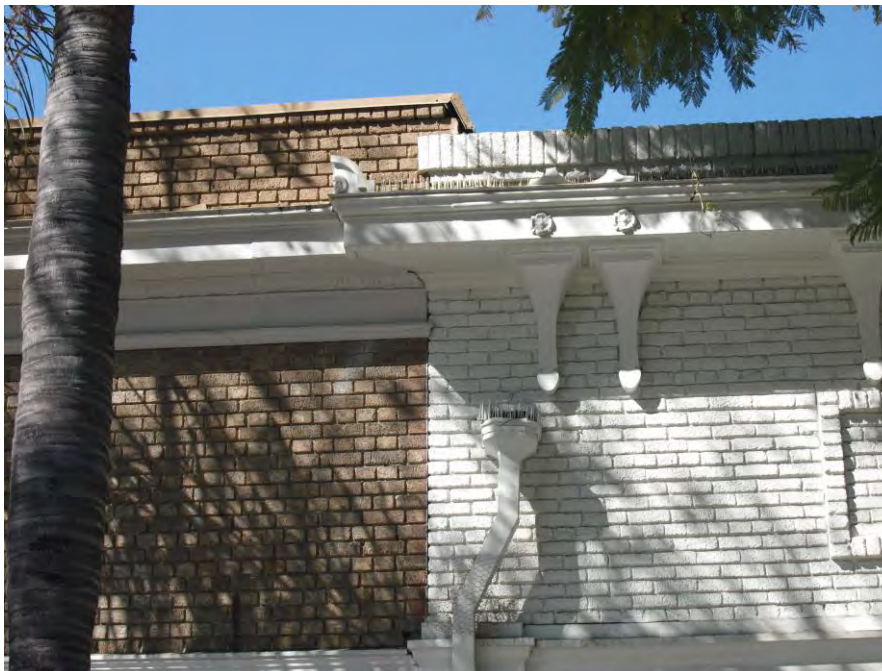
Detail view at South First Street, viewed facing west.
