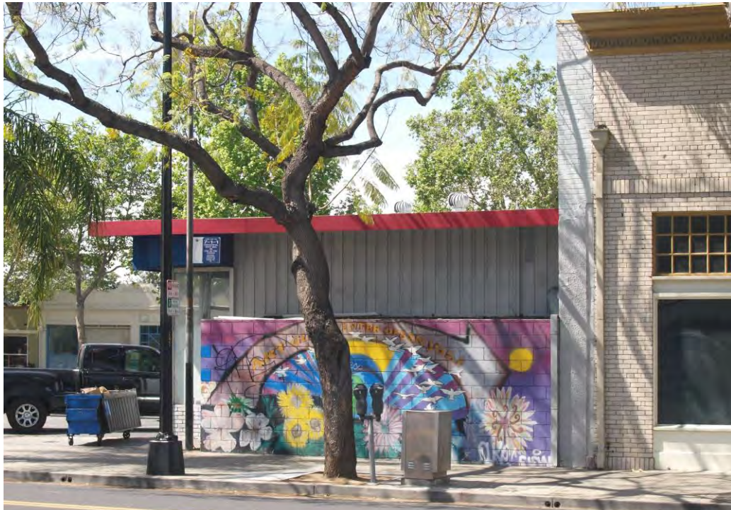
East side elevation, viewed facing west.
