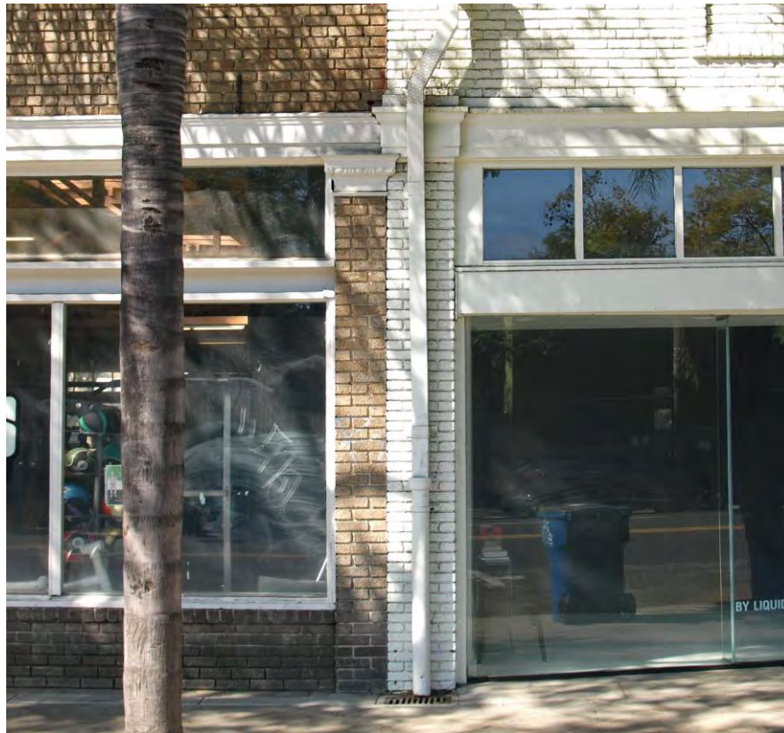
Detail view at South First Street, viewed facing west.
