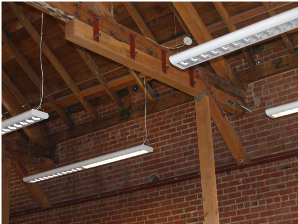
Internal structural reinforcements at internal wall and truss.
