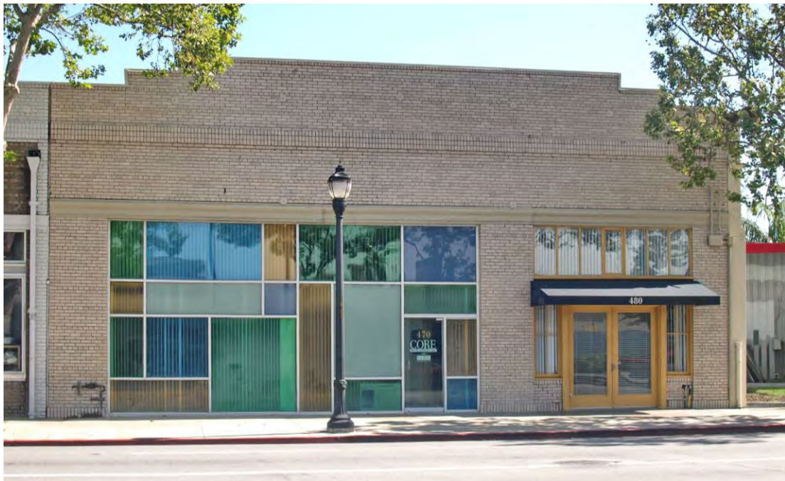
470-480 South Market Street, viewed facing east.
