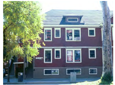
Fig 3-23 Historic structure on San Carlos Street.
