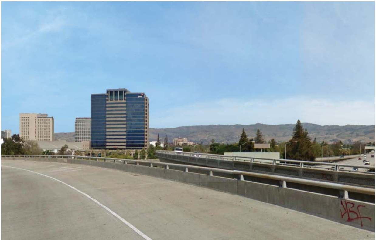
Existing - View of Downtown San José looking east from the southbound I-280 connector to northbound SR 87.
