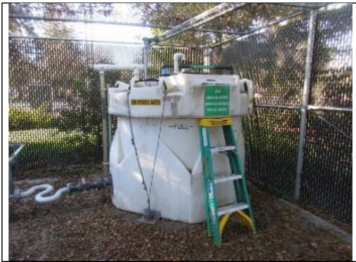
13. View of non-hazardous waste water tank in the enclosure adjacent to the west
