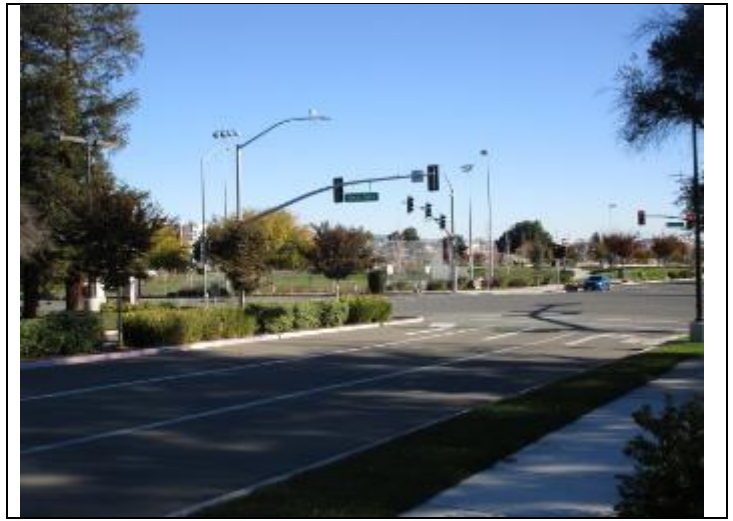
20. View of the intersection of Great Oaks Parkway and Charlotte Drive adjacent to the southeast
