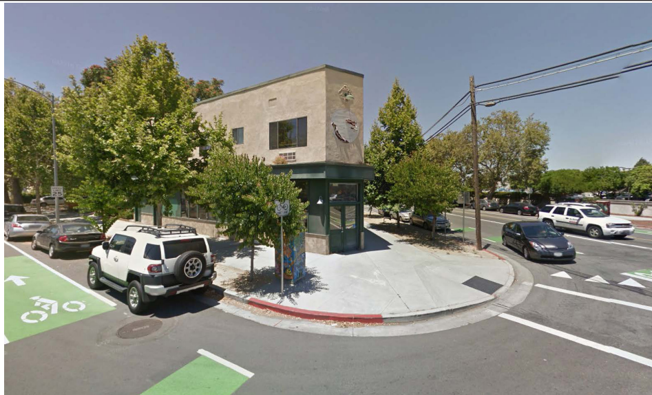
Photo 1. View of southeast portion of site looking northwest from Julian Street and Stockton Avenue.
