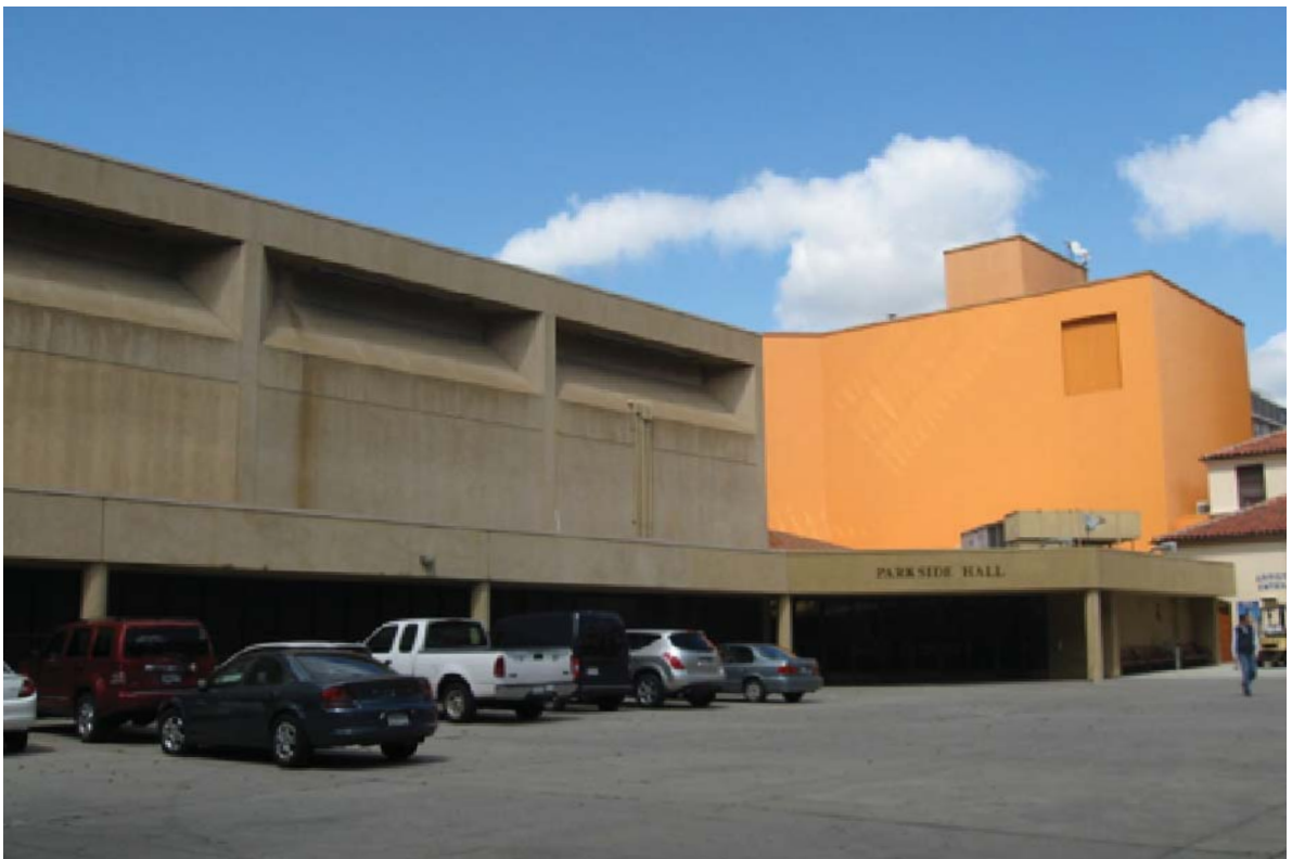
PHOTO 2: View of the truck loading area, looking east from the paseo.
