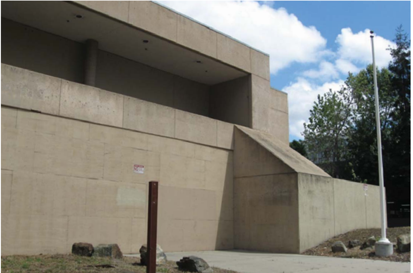
PHOTO 13: View of the surrounding development, looking southeast at the corner of Park Avenue.
