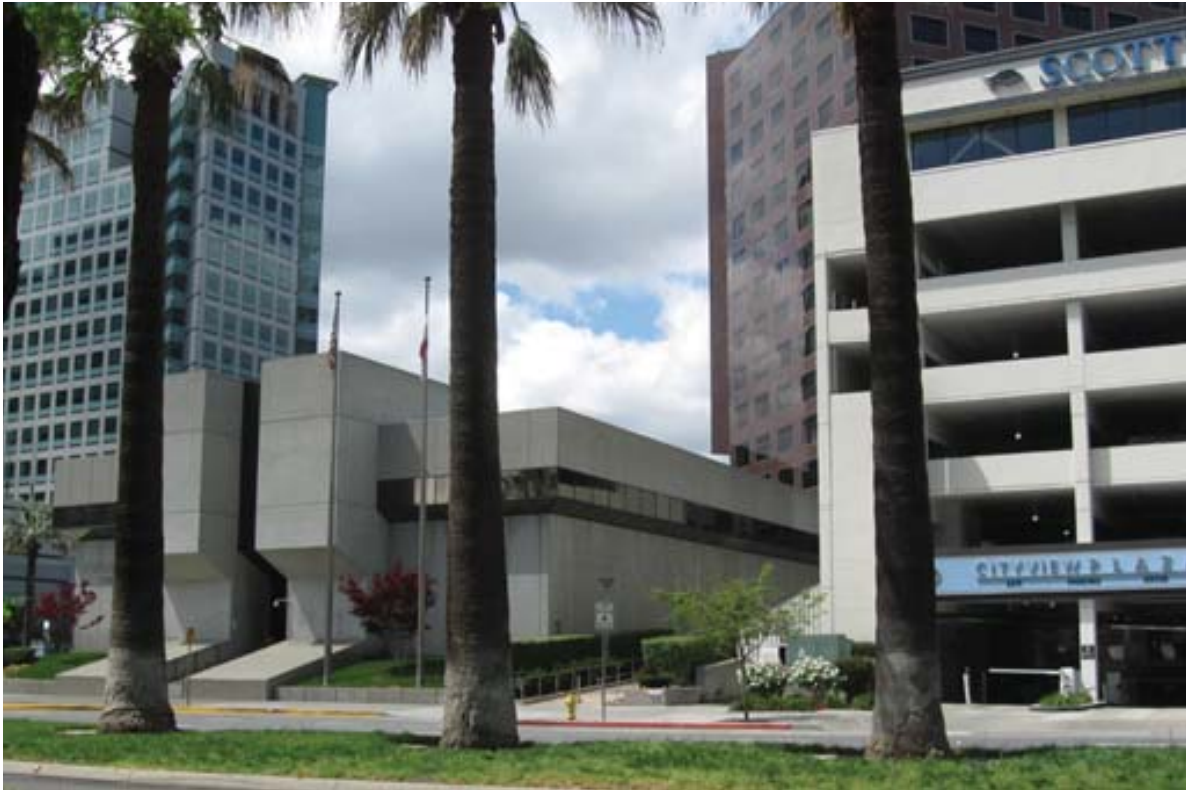
PHOTO 3: View of the westernmost building, looking northwest from Park Avenue.
