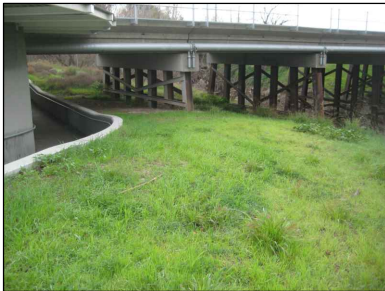
CURVE NORTH OF BRIDGE
