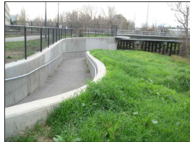
VIEW LOOKING SOUTH, BOTH RETAINING WALLS VISIBLE
