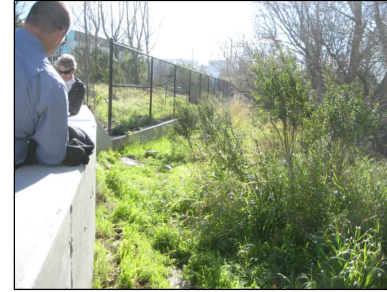
FENCE SOUTH OF UNDERCROSSING TRAIL
