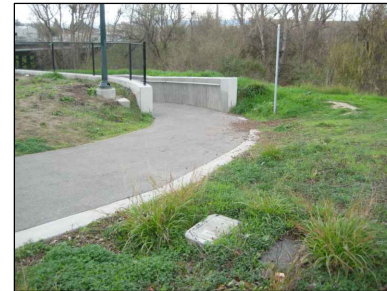
STARTING LOCATION OF RETAINING WALLS
