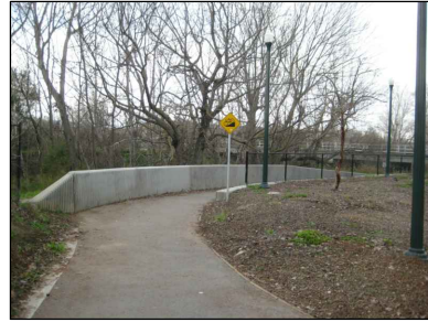
STARTING LOCATION OF RETAINING WALLS
