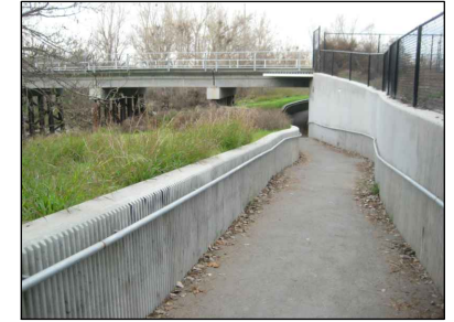
RETAINING WALLS AND RAILROAD BRIDGE
