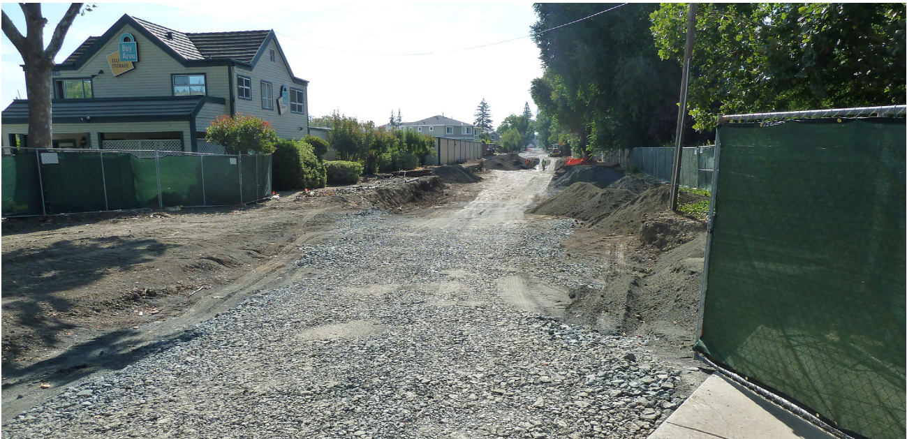
Photo taken during site clean-up
