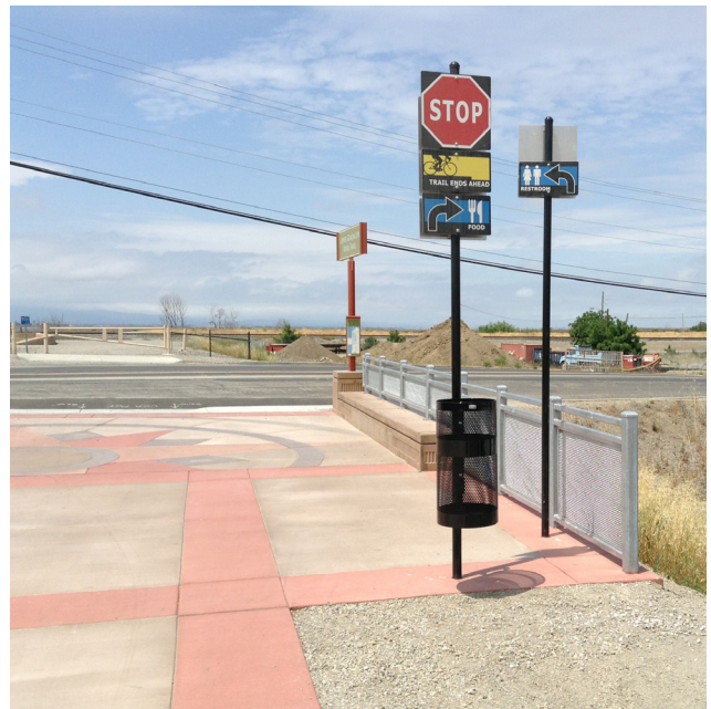
Example of San José trail with decorative paving with accent color, signage, and post-mounted waste receptacle.
