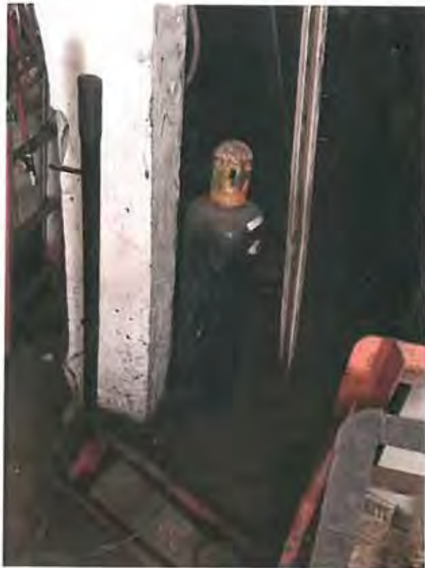
Photo 1. View of typical compressed acetylene gas container observed in the southern portion of the subject property building. Photograph taken August 16, 2017.
