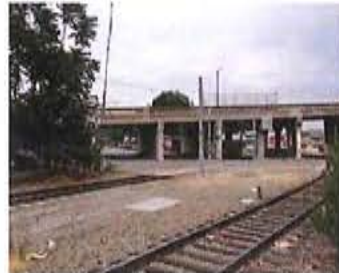
Site and Overpass from Rail Tracks
