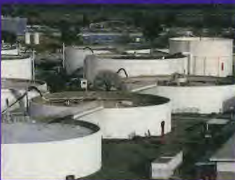
Digester Rehabilitation Project
