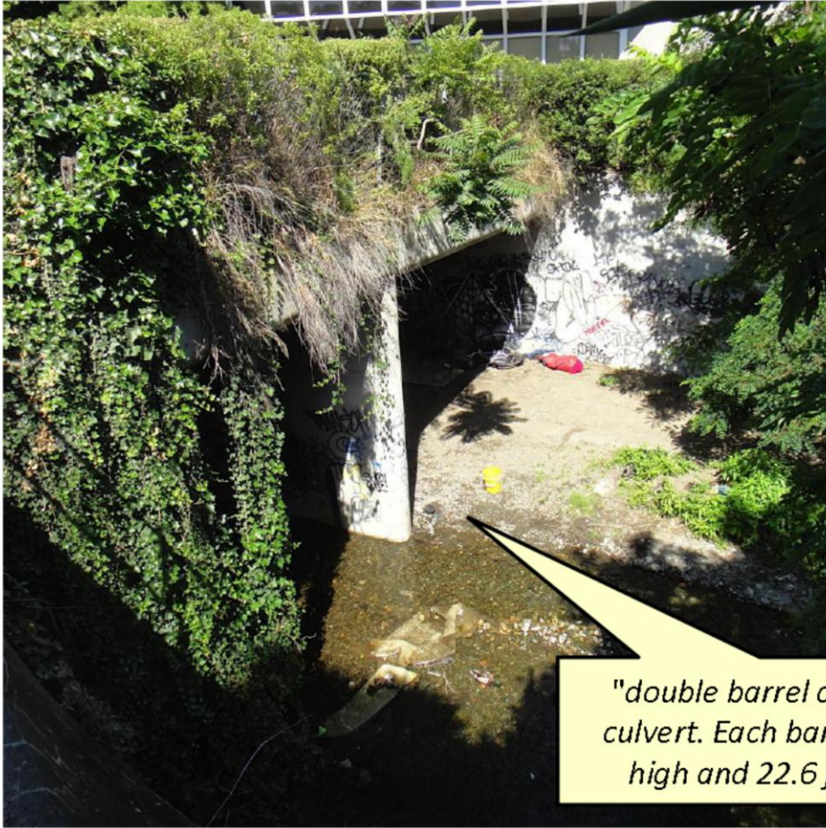
Fig. 4 – Northern End of the Los Gatos Creek Culvert
