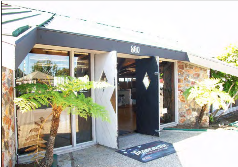
800 West San Carlos Street, former Cheim Lumber Company office and showroom. Main entrance. North façade, view southwest. LSA photograph, 5/6/14.
