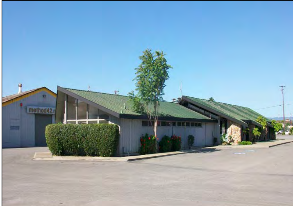
800 West San Carlos Street, former Cheim Lumber Company office and showroom. North and east façades, view southwest. LSA photograph, 5/6/14.
