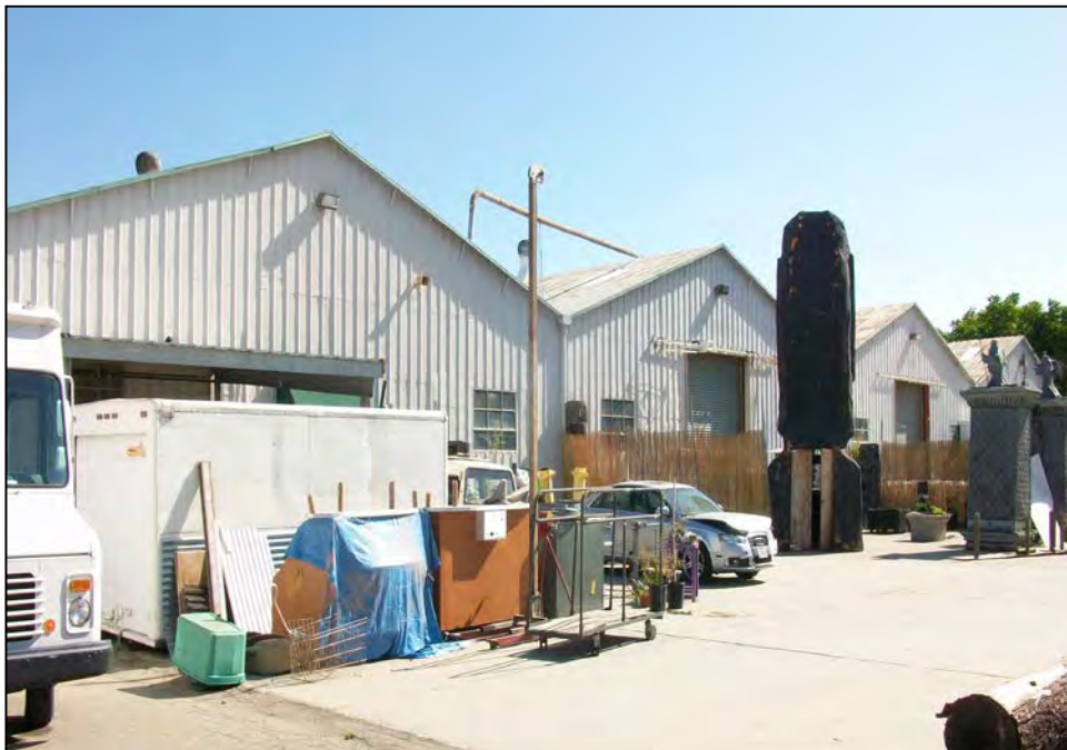
800 West San Carlos Street, former Cheim Lumber Company warehouse. South façade, view northeast. LSA photograph, 5/6/14.
