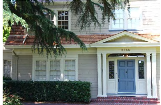
Wood shingle siding; Double-hung multi-lite wood sash windows, some grouped in pairs and tripartite configurations.
