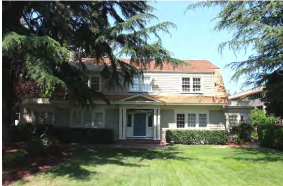
Two story massing and rectangular footprint with square footprint one-story side wings; side gambrel roof with long shed dormers.
