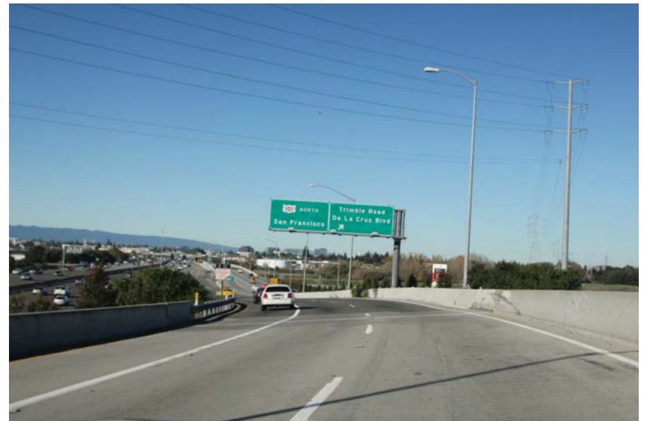
Northbound SR 87 Ramp - Property 10 & 11
