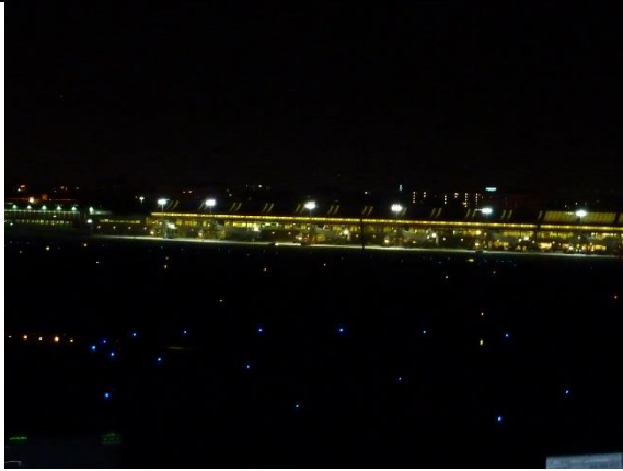
Airport Pole Lighting Inside Tower – 63 Nits
