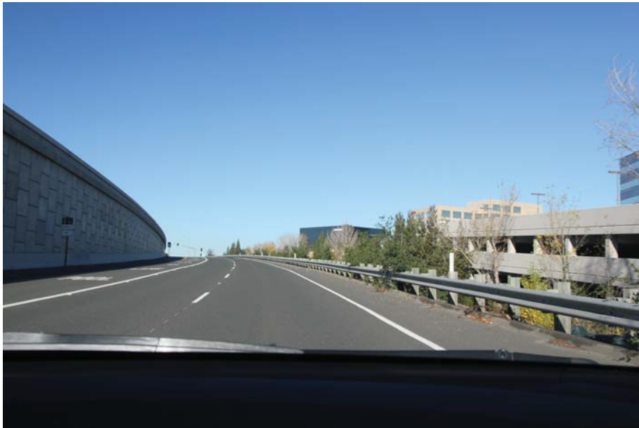
Northbound Skyport Ramp - Property 15
