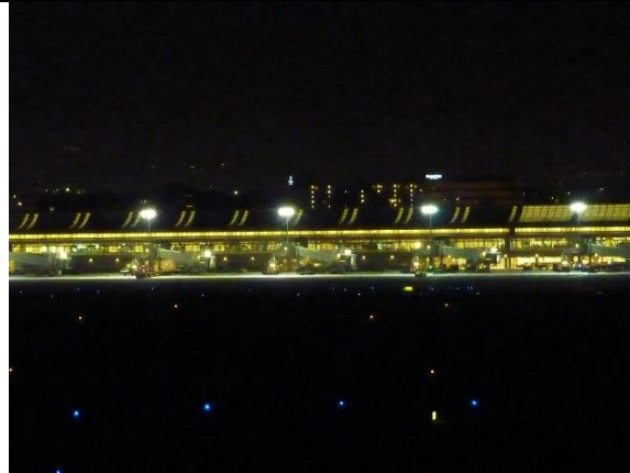
Airport Pole Lighting Outside Tower – 72 Nits
