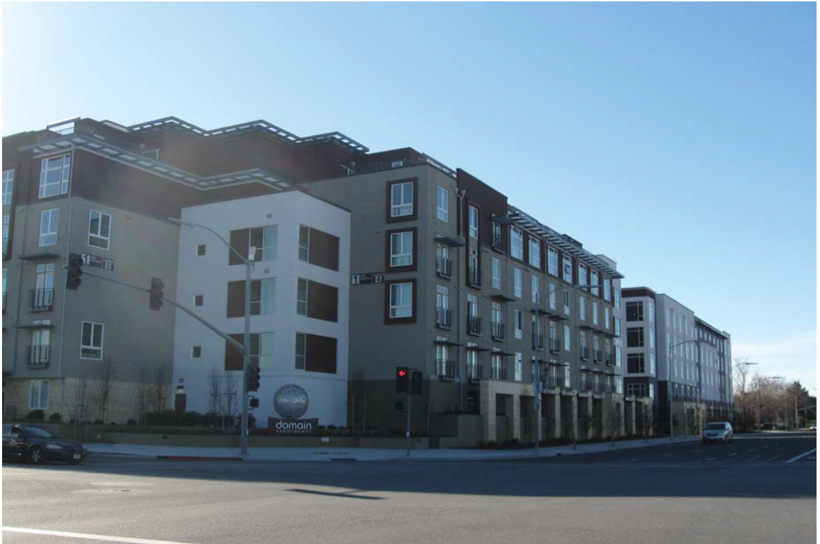
PHOTO 1: Northbound N. 1st Street, at the N. 1st Street/Headquarters Drive intersection.
