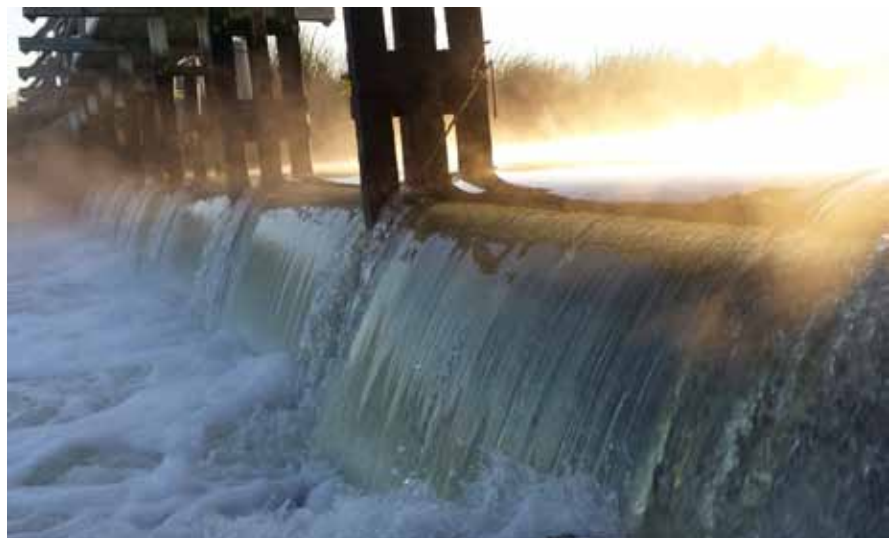
Outfall at the San José-Santa Clara Regional Wastewater Facility
