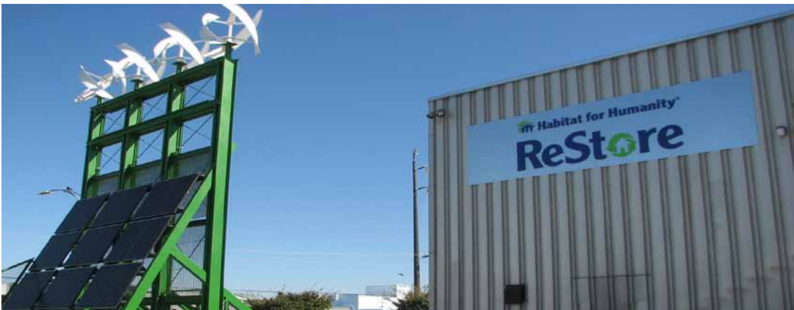
Wind turbine and solar installation at the Environmental Innovation Center, featuring Habitat for Humanity ReStore, Prospect Silicon Valley, and Santa Clara County Household Hazardous Waste facility, as well as office, meeting and event space.
