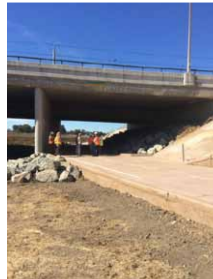
Tasman Drive Undercrossing
