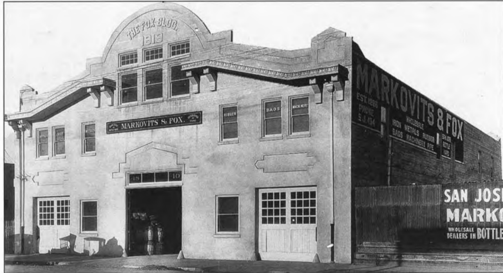
Markovitz and Fox had operated a successful scrap and salvage company in San Jose since the late 19th century. In 1919 they erected this building at 40 North Fourth Street.
