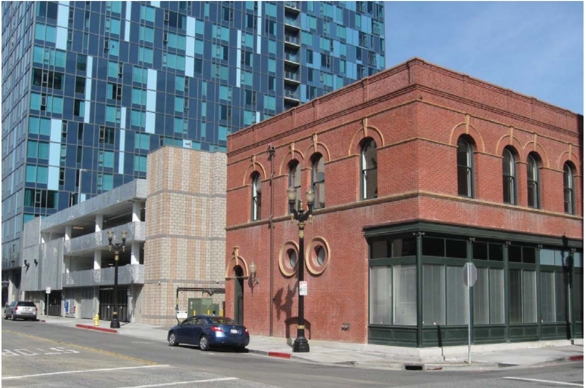
PHOTO 7: View of the Sunol Building, looking northeast from Post Street.
