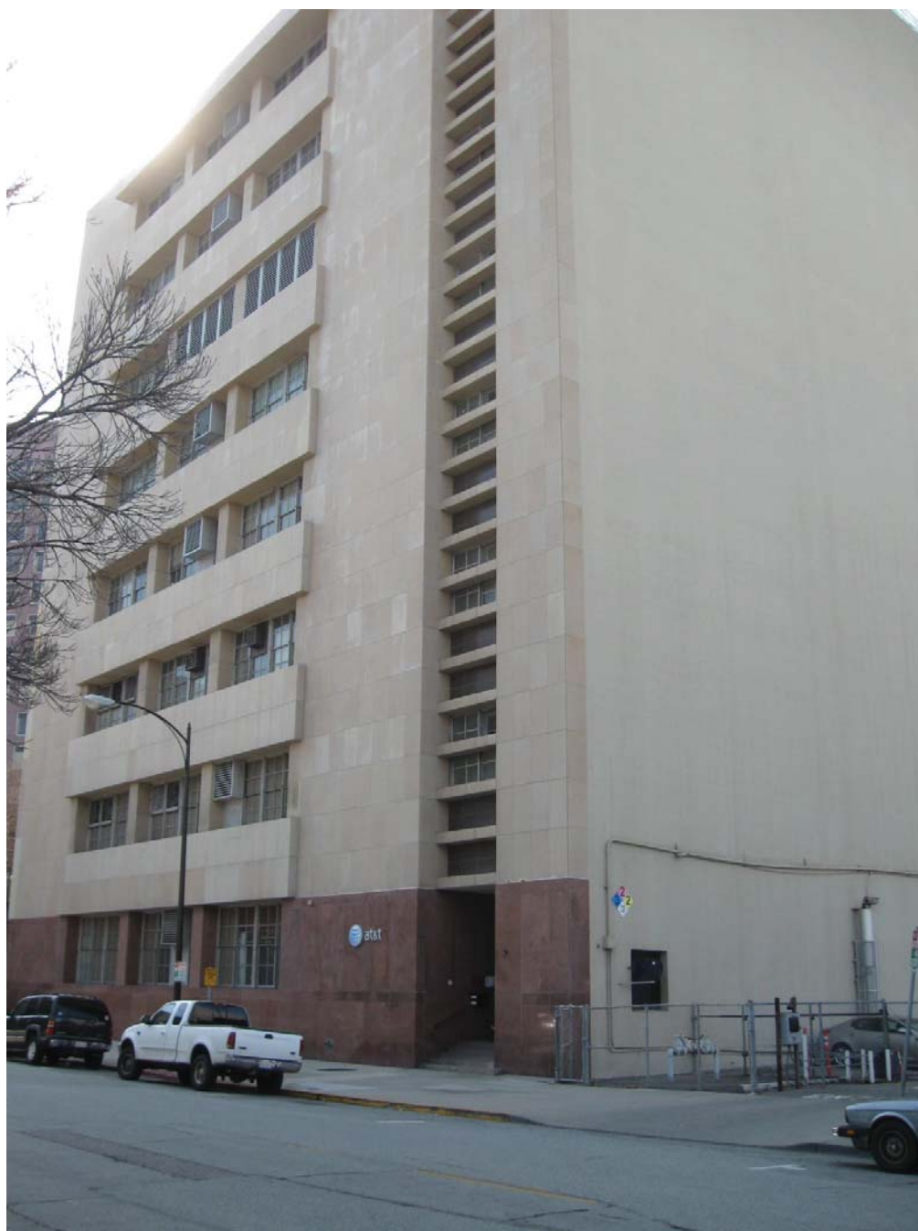
PHOTO 9: View of the AT&T Building, looking south from the project site.
