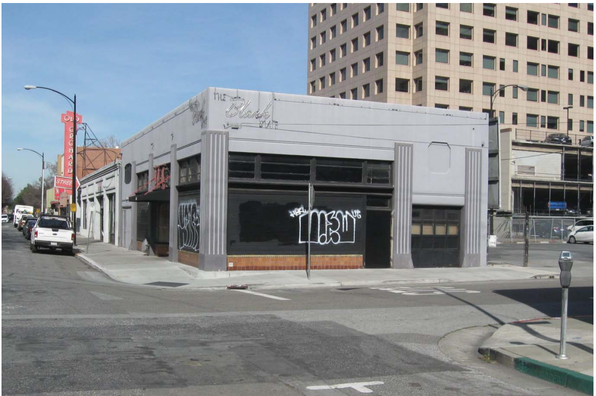
PHOTO 8: View of the Berger Building, looking north from S. Almaden Avenue.
