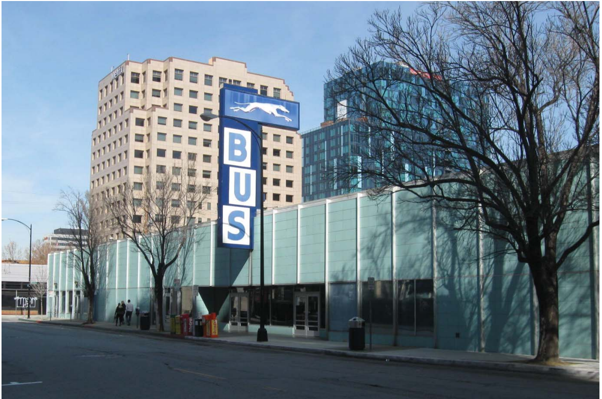
PHOTO 1: View of the existing bus station, looking northeast from South Almaden Avenue.
