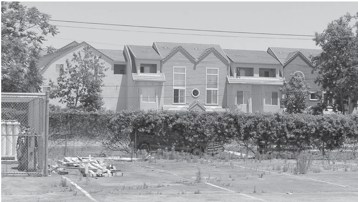
Photo 6: View east from within the Corporation Yard site
