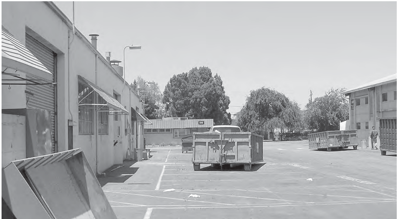
Photo 1: Corporation Yard site
