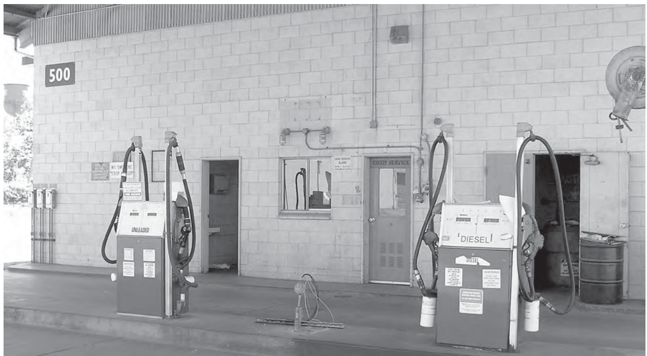
Photo 2: Fueling area on Corporation Yard site
