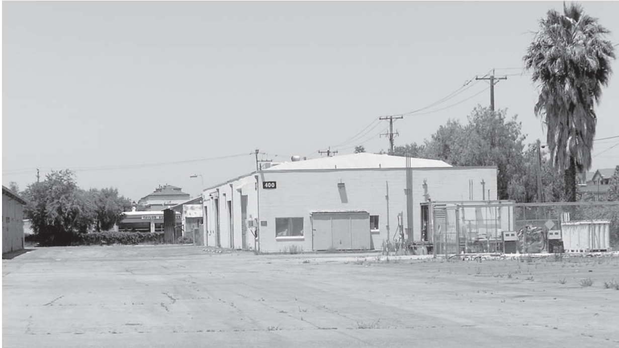
Photo 5: View north from within the Corporation Yard site
