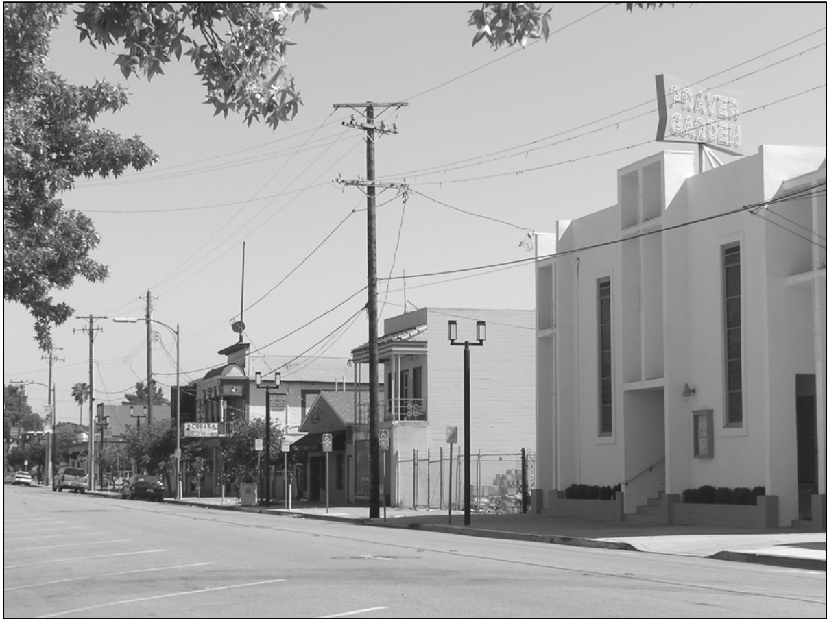
Photo 1: View southwest of building on west side of North 6th Street.
