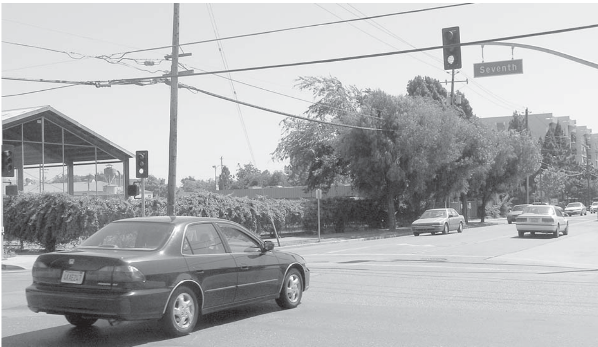
Photo 4: View of Corporation Yard site, looking west from the intersection of North 7th Street and Taylor Street
