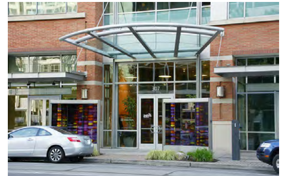
▼ Well-defined entrance for residential/mixed-use buildings
