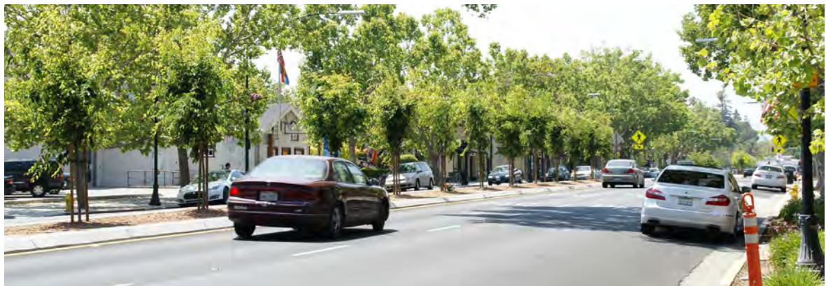
Median landscaping as part of the improvements along The Alameda
