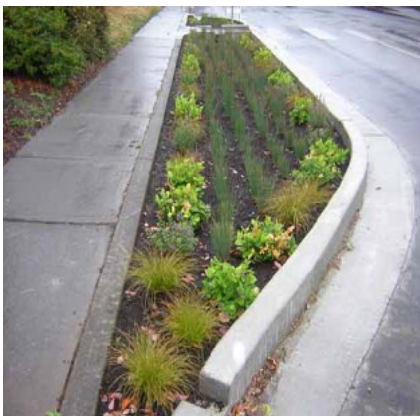
Rain gardens and infiltration planters can be used to mitigate stormwater runoff.
