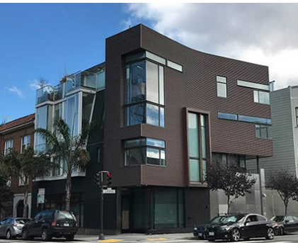
Well-defined corner elements by recession, or projection, differentiation in height, transparency, and building materials. These corner elements make the entrance to the building identifiable, inviting, and human scale by breaking up the massing of the building.
