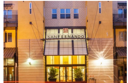
Well-defined entrance for residential/mixed-use buildings
