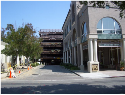
Entrances to loading and service areas shall be from side streets or alleys where possible.
