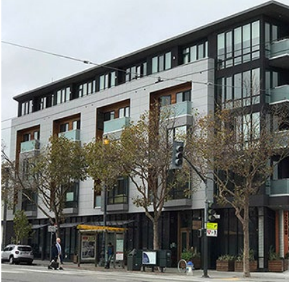
Three parts of a building, base, middle, and top, is evident in the buildings below. Projection and recession in facades, variations in the height, projected or recessed balconies, and awnings help to break down the scale of a building.
