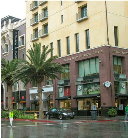
Ground floor retail, differentiated from the upper floors by a change in color, materials, and recessed storefronts that are separated from each other.
