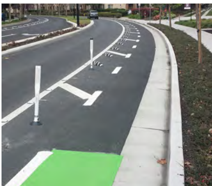
Protected bike lanes (Class IV bikeway) includes vertical separation such as delineations (pictured above).
