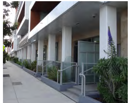
The top photo shows active uses that attract foot traffic, while the bottom photo shows private uses. Both frontages, however, feature transparency and pedestrian-oriented design.
