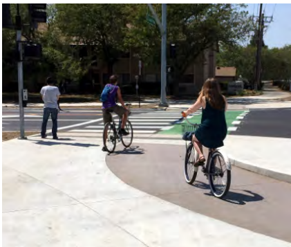
A Dutch-style intersection delineates uses and creates safer crossings for people who walk and people who bike.
