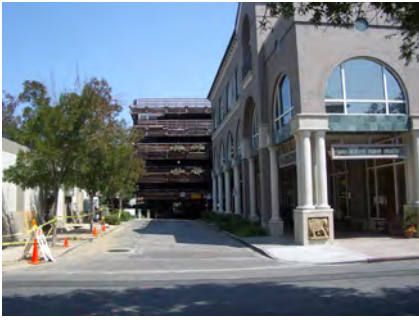
Entrances to loading and service areas shall be from side streets or alleys where possible.
