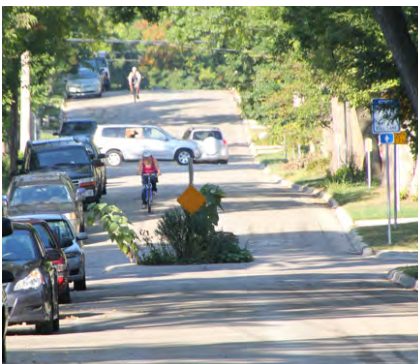
Chicanes can be effective in calming vehicular travel speeds and improving safety for all people of the road.
