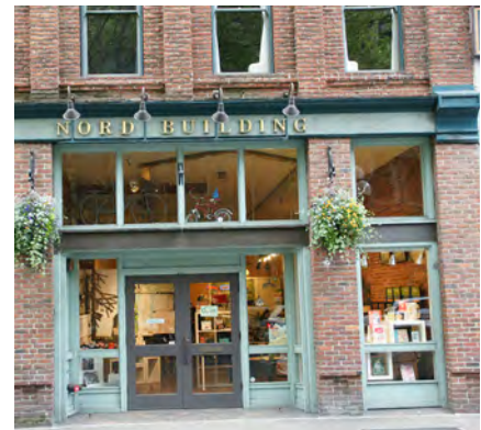
Traditional storefront design displaying merchandise at two levels, transparent facade, inviting entrance, ornamental planting box and interesting use of store front lights and signs.
