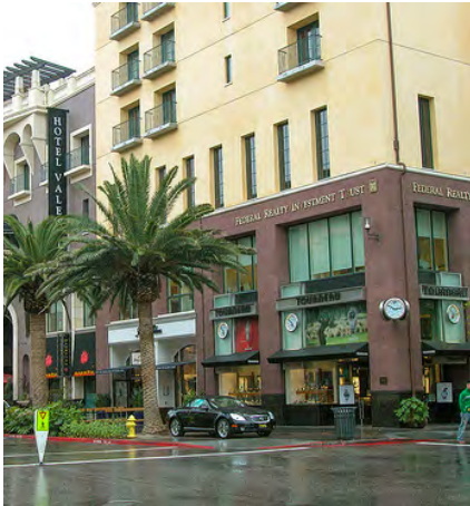
Ground floor retail, differentiated from the upper floors by a change in color, materials, and recessed storefronts that are separated from each other.
