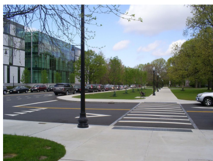
Mid-block crossings can provide direct routes and can enhance safety for people who walk.
