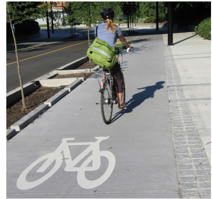
Class IV cycle tracks are separated from vehicular and pedestrian uses and are proposed on major streets in the Urban Village area where appropriate.
