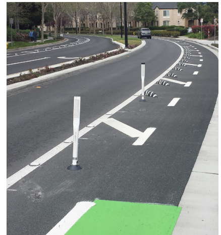
Protected bike lanes (Class IV bikeway) includes vertical separation such as delineations (pictured above).
