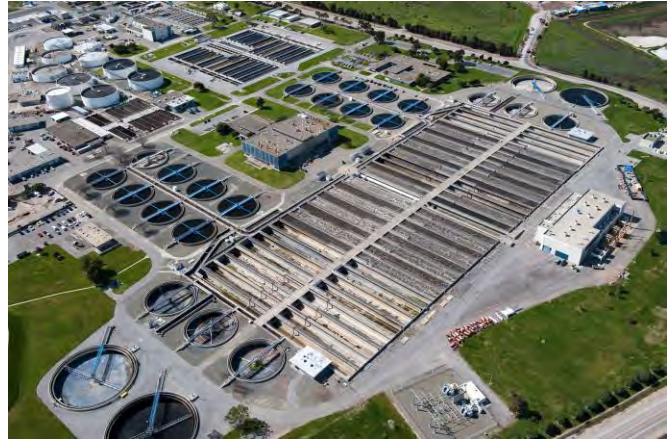
San José-Santa Clara Regional Wastewater Facility
