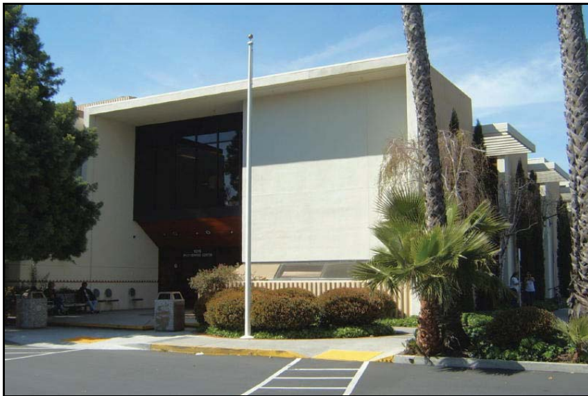
Corporate Modern variant, located at 1075 East Santa Clara Street (SNI 6), and expressed as large volumes of concrete set within a plaza off of the street. Photo: PAST Consultants, LLC
