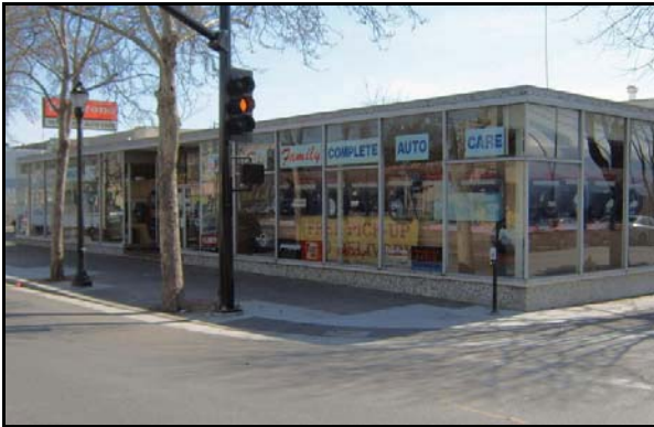
This Commercial Modern building at 477 South Market Street (SNI 11) displays wide expanses of glass and a ceramic tile base. Photo: PAST Consultants, LLC
