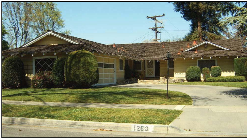
Custom ranch house on Norval Way. Known as the California Ranch Style, this low-slung house features a rambling plan with generous picture windows, a prominent front garage, wood roof shingles and stone cladding at the base. Photo: PAST Consultants, LLC
