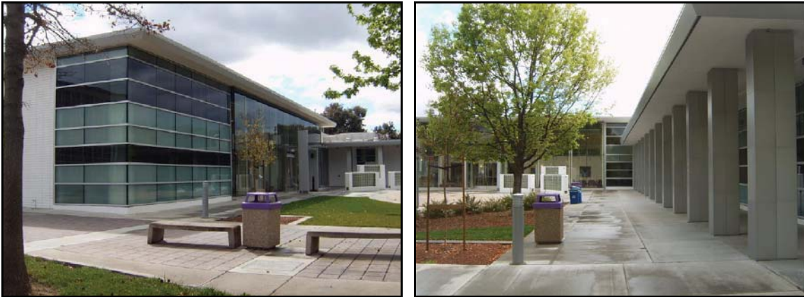
Two views of the Student Service Center Building (1962) at San José City College (SNI 2). Photos: PAST Consultants, LLC
