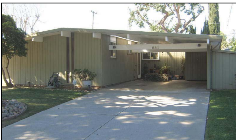
Post-and-Beam Style house on Richmond Avenue (SNI 2). Note the projecting wood beams and low-slung roof. Photo: PAST Consultants LLC
