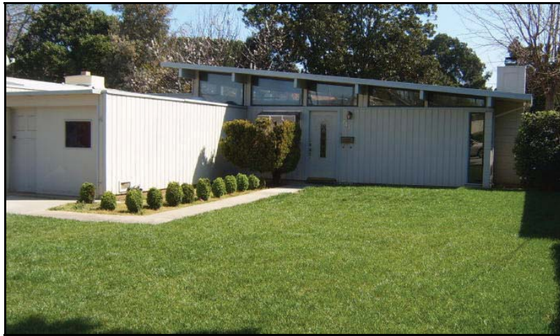
Post-and-Beam example on Richmond Avenue (SNI 2). In this case, the structural module permits an exposed bank of clerestory windows, framed by the exposed roof beams. Photo: PAST Consultants LLC
