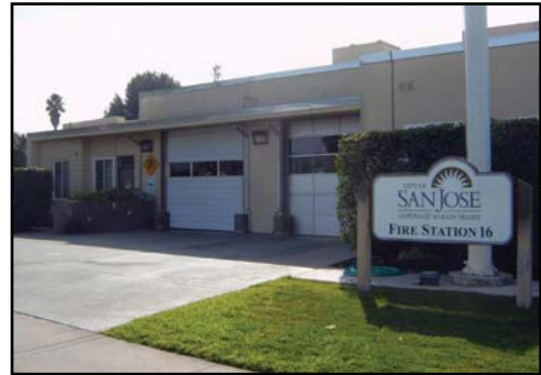
Fire Station No. 16, 2001 S. King Rd. (SNI 10) Photo: PAST Consultants, LLC
