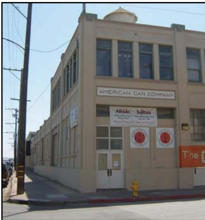
Example of an extant canning facility: The American Can Company at Fifth and Martha streets (SNI 13). Photo: PAST Consultants, LLC
