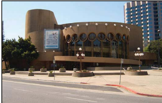
Center for the Performing Arts (1972, Candidate City Landmark), designed by Taliesin Associated Architects, in the Organic Style. Photo: PAST Consultants, LLC
