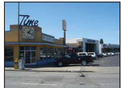
349 South Bascom Avenue (SNI 2) Photo: PAST Consultants, LLC
