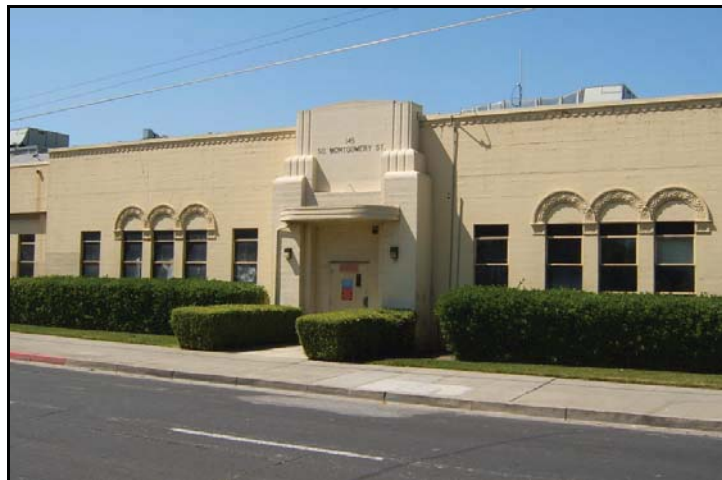
Industrial building completed in the late 1930s for the Sunlite Baking Company at 175 South Montgomery Street (SNI 2). Streamline Moderne details include the horizontal cornice band and ribbon windows, contrasted by the projecting, stepped front entrance capped by a canopy with rounded corners. Photo: PAST Consultants, LLC
