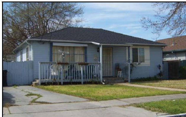
Early Minimal Traditional House on Balboa Avenue (SNI 7), featuring a hipped roof with shallow eaves, window shutters, and a simple front porch on slender columns of dimensional lumber. Photo: PAST Consultants, LLC
