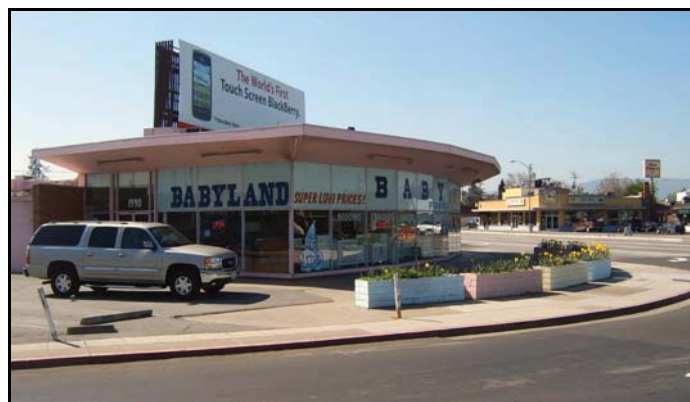
Commercial Modern adaptation to a curved corner site, at intersection of West San Carlos Street and Bascom Avenue (SNI 2). Photo: PAST Consultants, LLC
