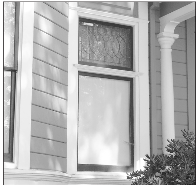
Typical double-hung window components.
