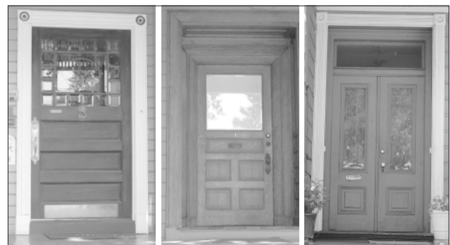
Preserve the functional and decorative features of original windows and doors.
