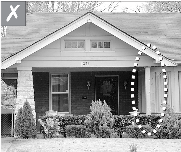
Preserve an original porch. Avoid using a porch support that would be substantially smaller than other supports on the porch or than seen historically.
