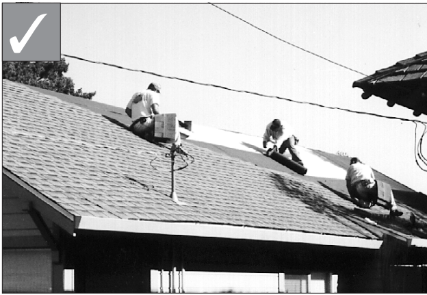
Composition shingles are an acceptable roofing material. (Napa, CA)
