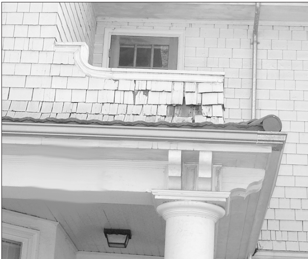
Do not remove damaged materials that can be repaired.
