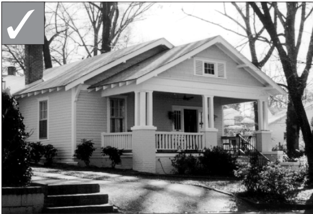
When reconstructing a porch, use supports that are of adequate size. The design of this porch was based on neighboring buildings of similar character and age. (Spartanburg, SC)
