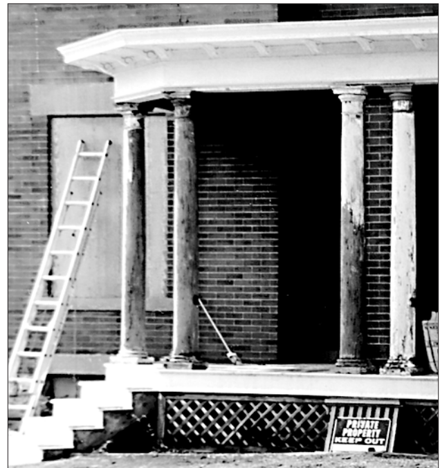
Repairing rather than replacing porch elements always is the preferred approach.
