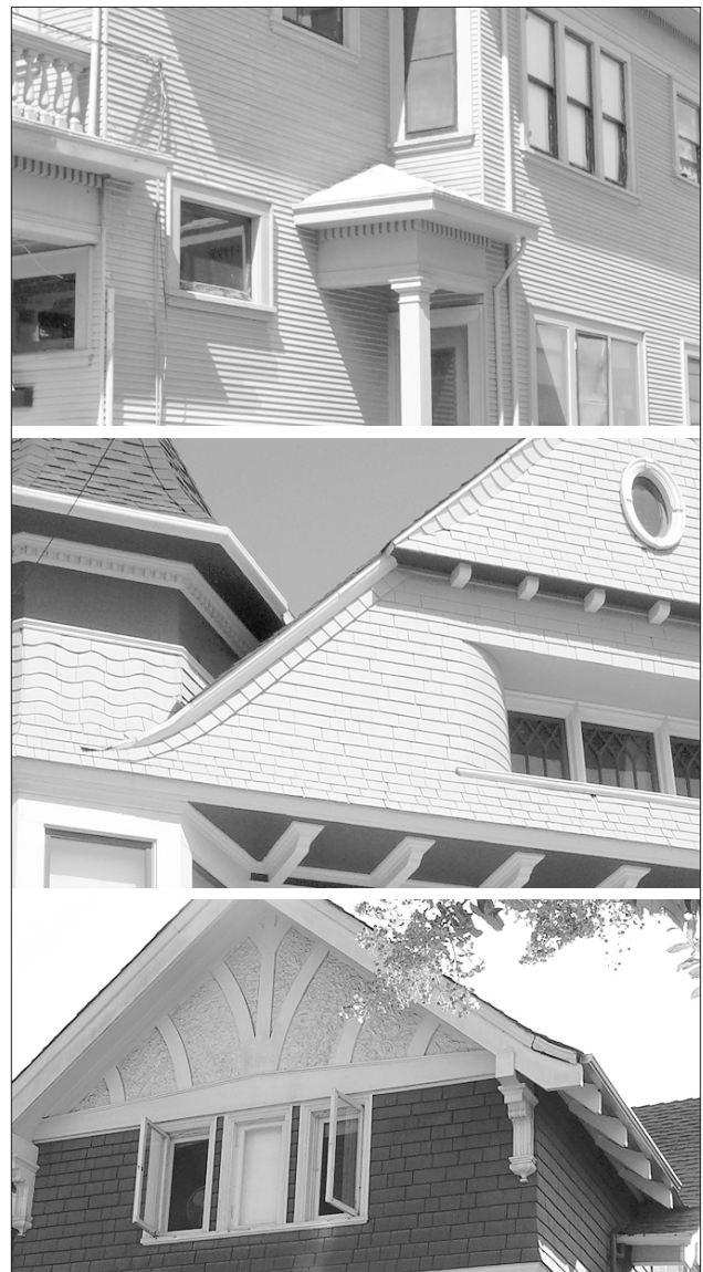
Retain and preserve original wall and siding materials.
