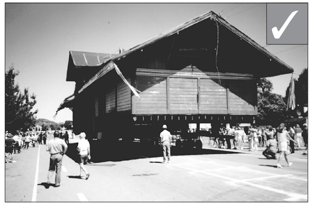
Before a building is moved, a plan must be in place to secure the structure, provide a new foundation and to restore it. (Danville, CA)
