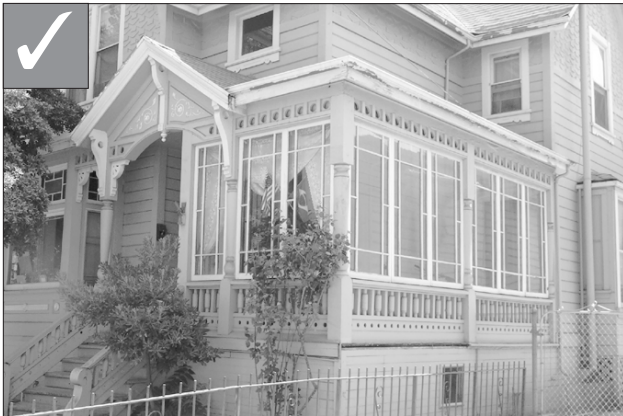
Where a porch must be enclosed, use transparent materials and place them behind the balusters and balustrade to preserve the visual character of the porch.
