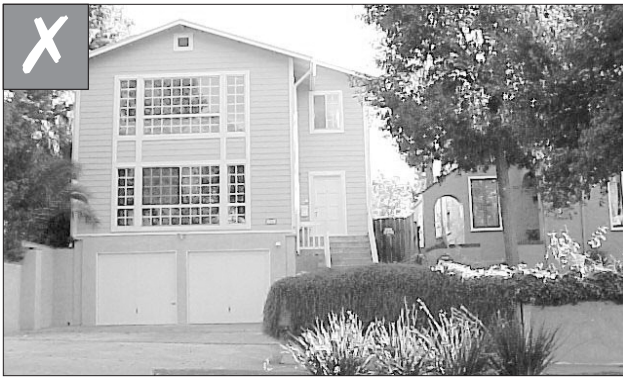
Although some buildings and their entrances were raised a few feet traditionally, a first floor or entrance that is raised an entire story—to accommodate a garage—is inappropriate. (Pasadena, CA)
