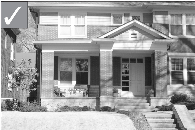
Using contemporary interpretations of historic styles is encouraged for new buildings. (Memphis, TN)
