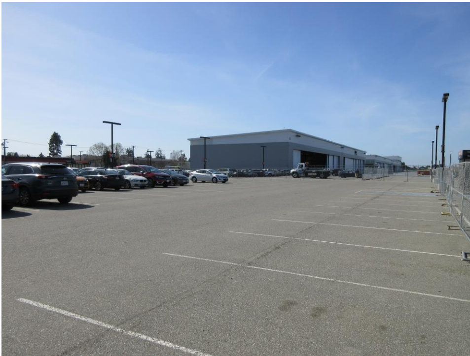
Photo 1: View of Project site looking to the north from the southerly border with the existing FBO hangars in the background.
