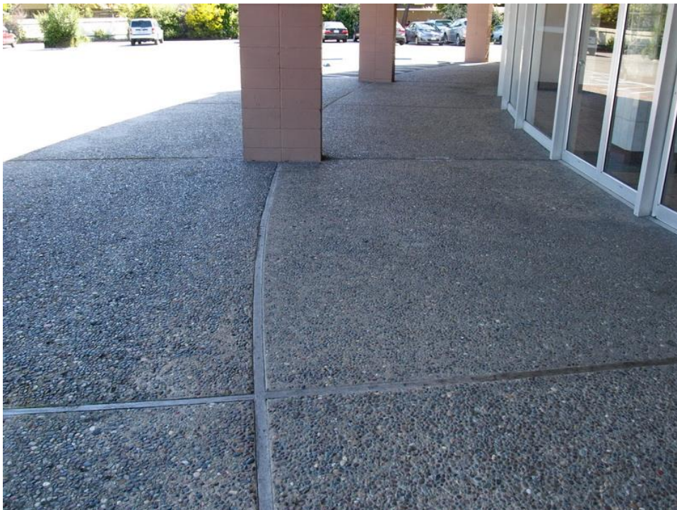
Aggregate concrete sidewalk at entry, viewed facing east.
