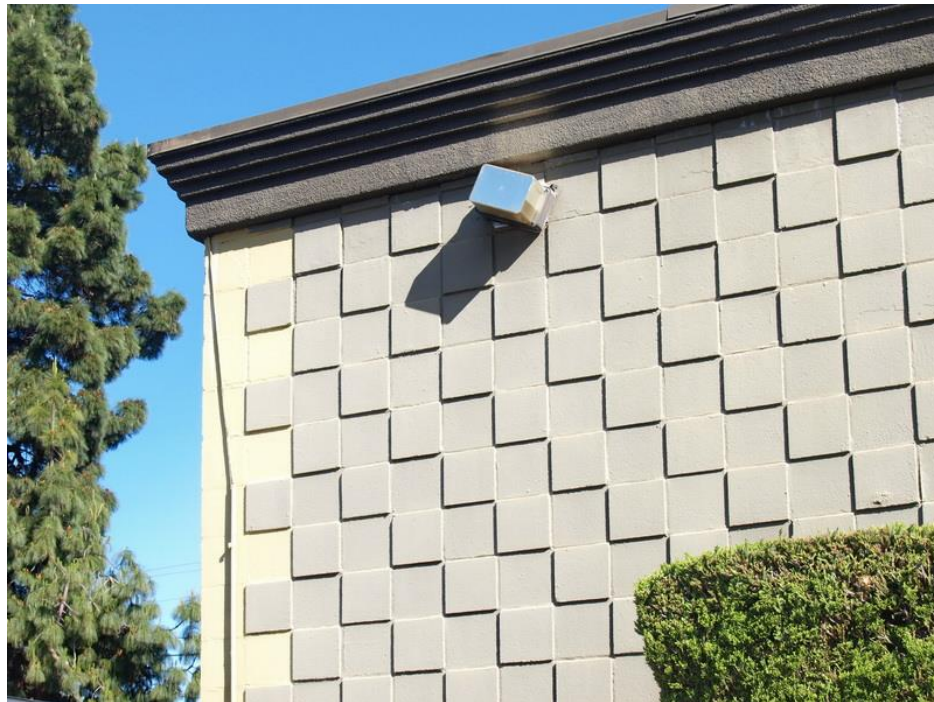
Roof detail at southwest corner, viewed facing northwest.
