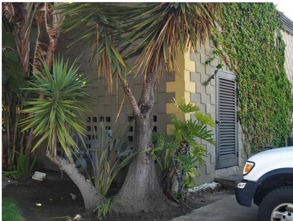
Detail at northwest corner, adjacent to rear parking, viewed facing southeast.
