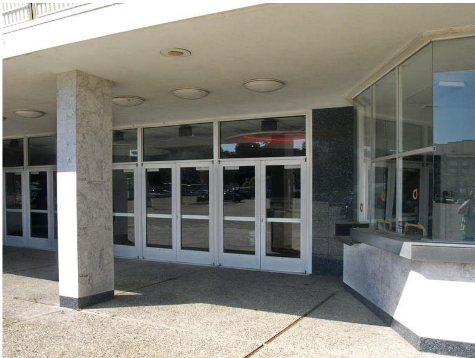
Entrance to lobby, viewed facing southwest.
