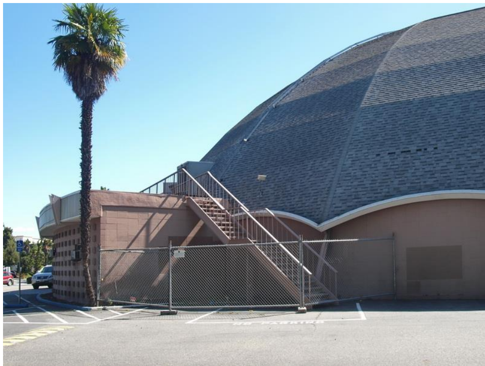
West side second story exit stairs, viewed facing northeast.
