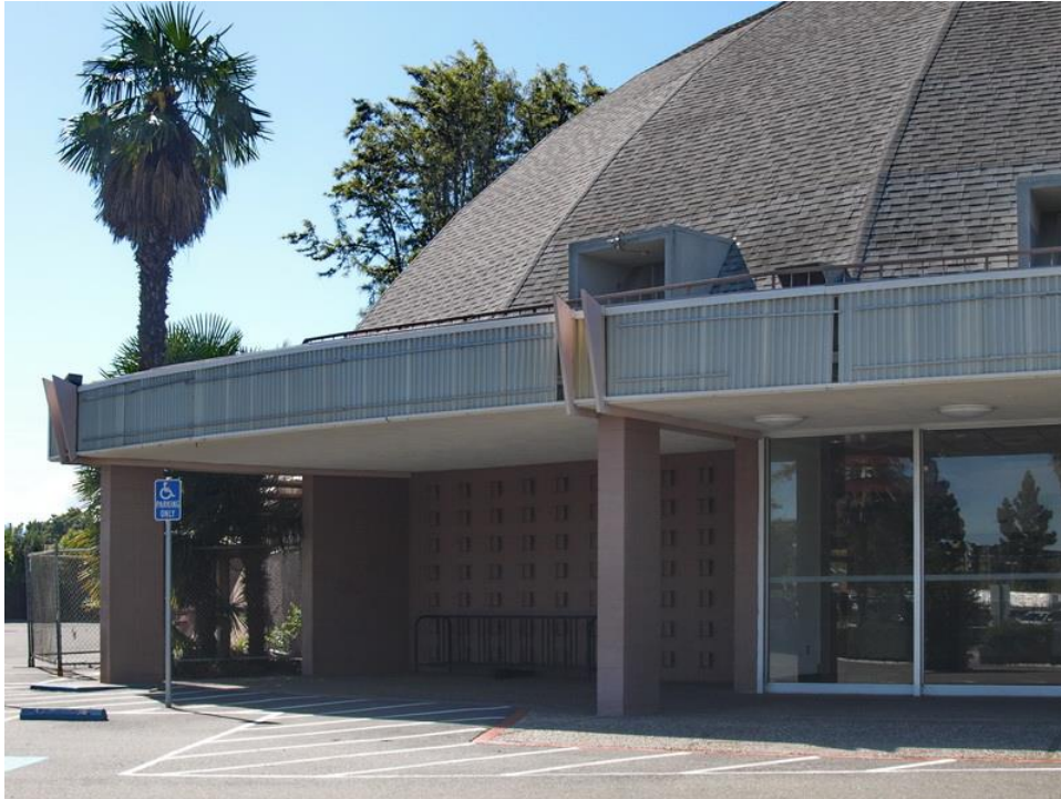
Second story exits above marquee, viewed facing southwest.
