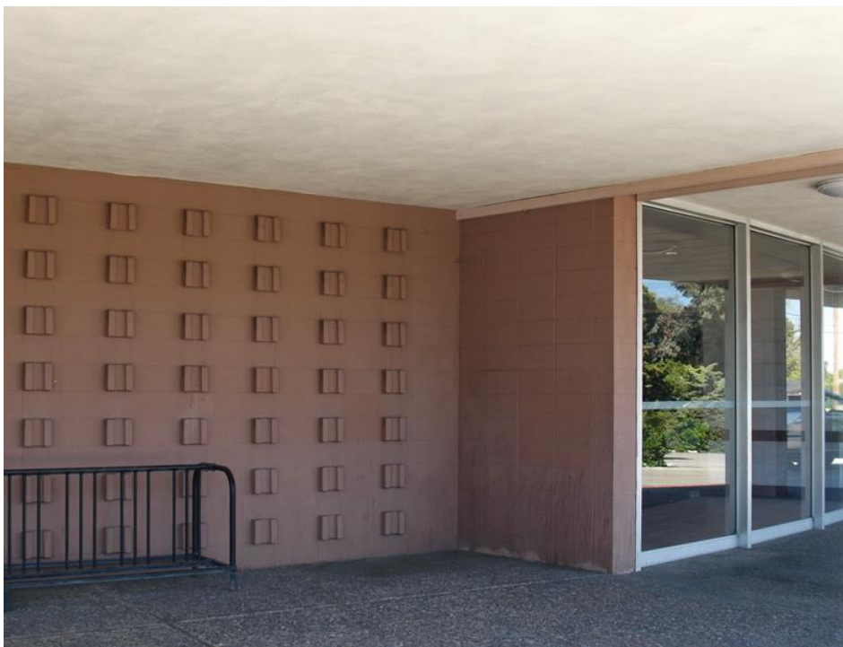
Wall detail, adjacent to lobby entrances, viewed facing southwest.
