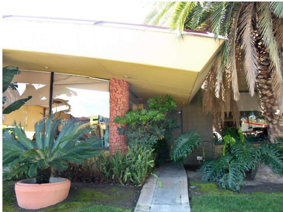
Eave detail, viewed facing south.
