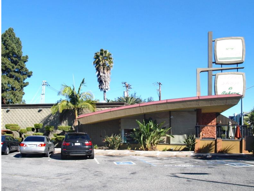
South elevation, adjacent to parking lot, viewed facing north.
