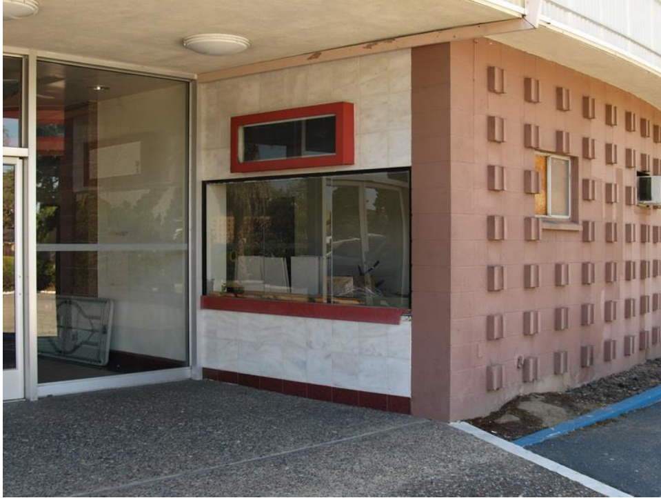
Ticket window adjacent to front entrance, viewed facing southwest.
