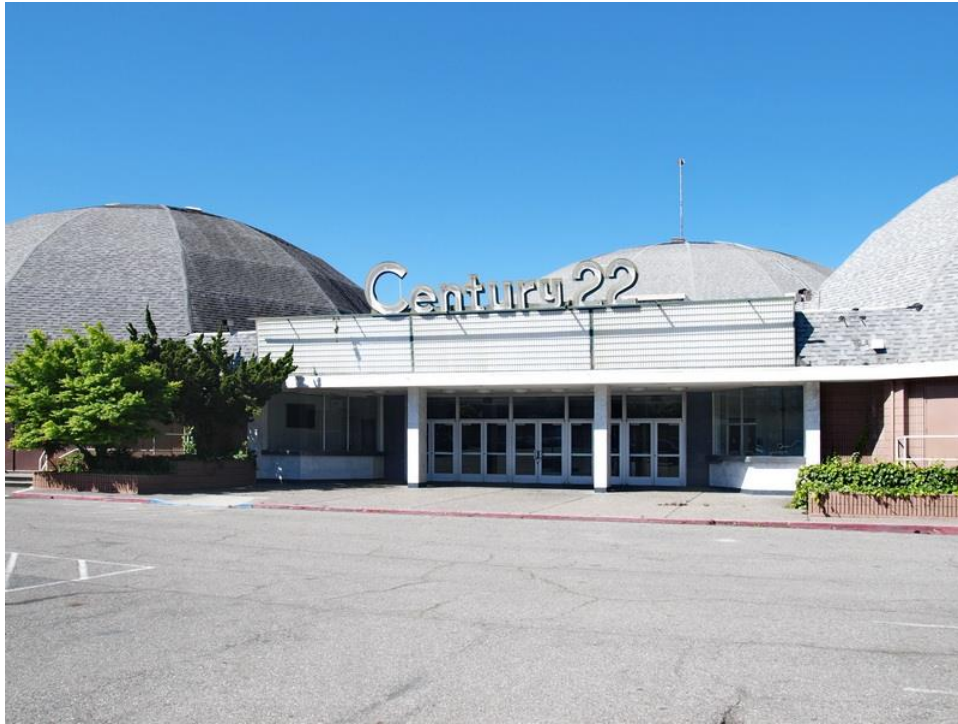
Front elevation, viewed facing west.
