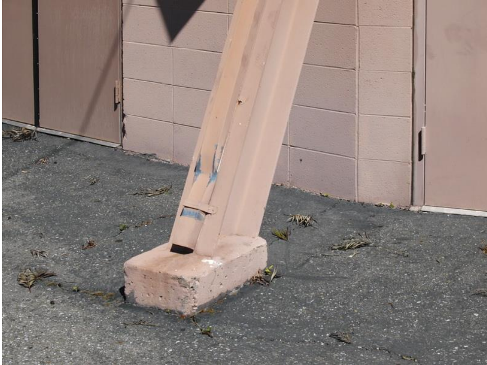
Roof brace detail at ground level.
