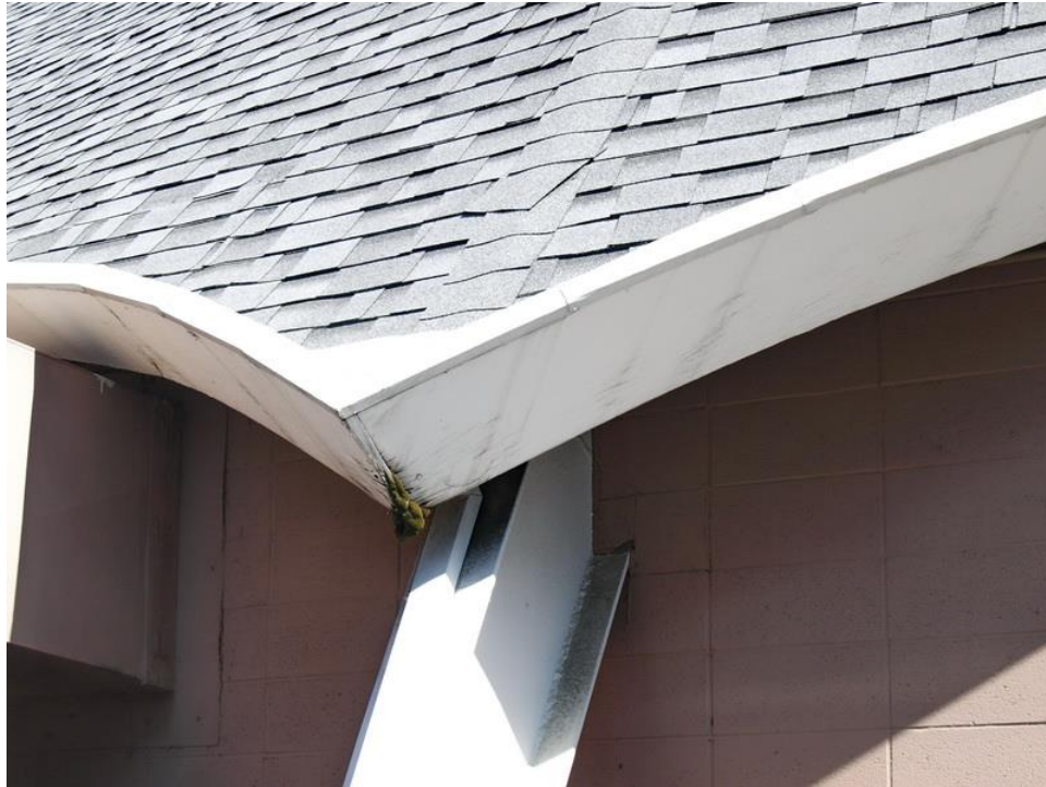
Curved or scalloped eave and brace detail.
