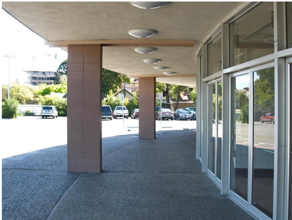
Entrance gallery, viewed facing east.
