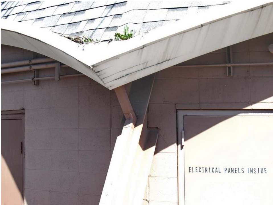
Eave and bracing detail.
