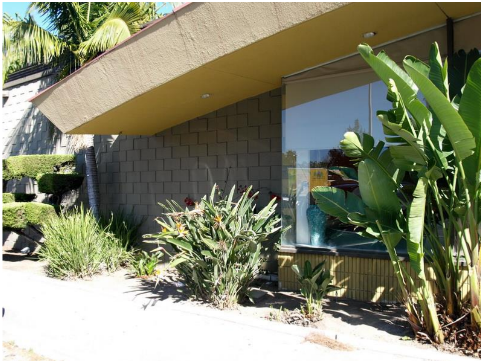
South façade, roof and wall detail, viewed facing northwest.
