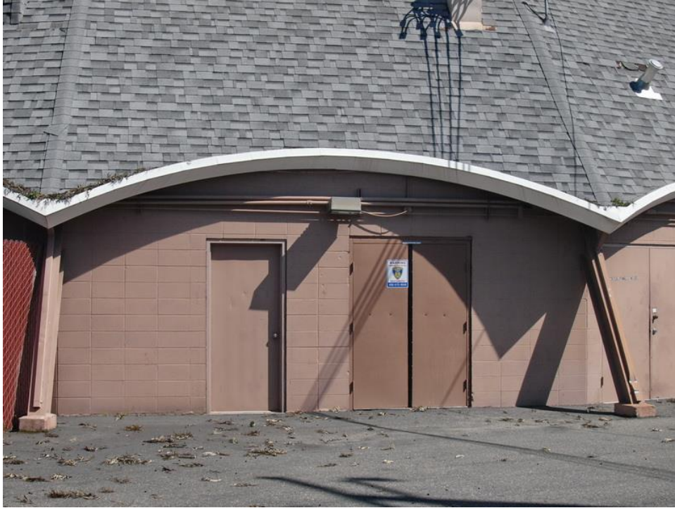
Curved or scalloped eaves and bracing.
