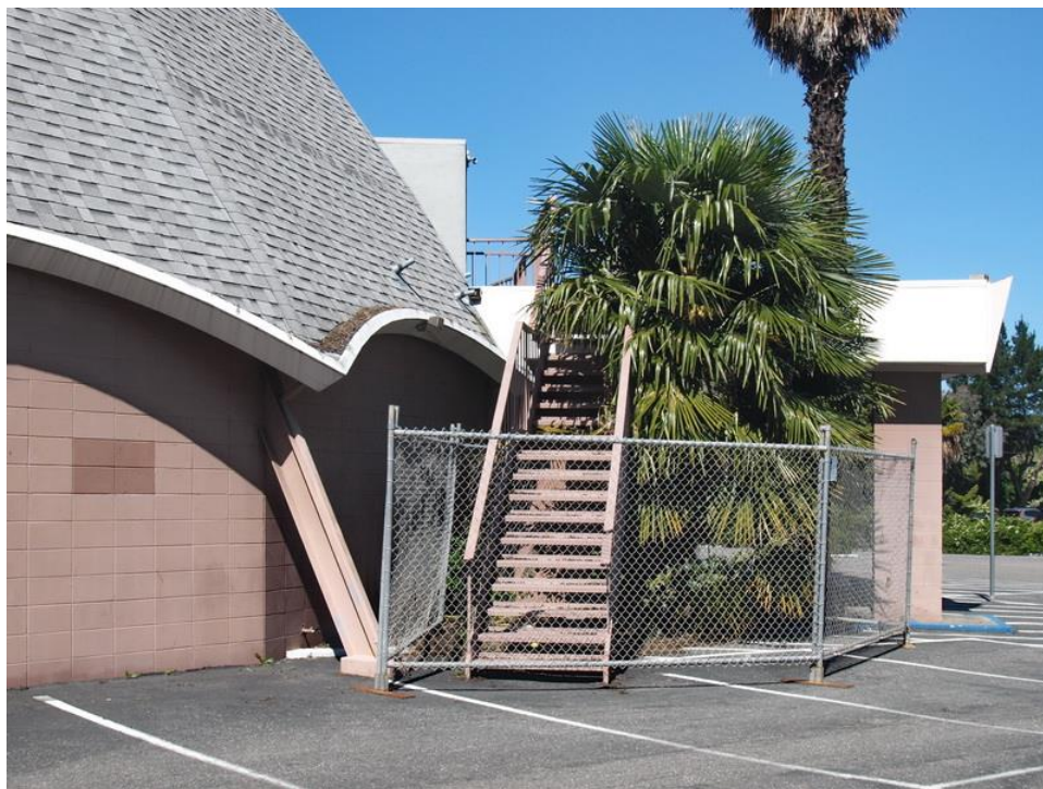
East side second story exist stairs, viewed facing northwest.
