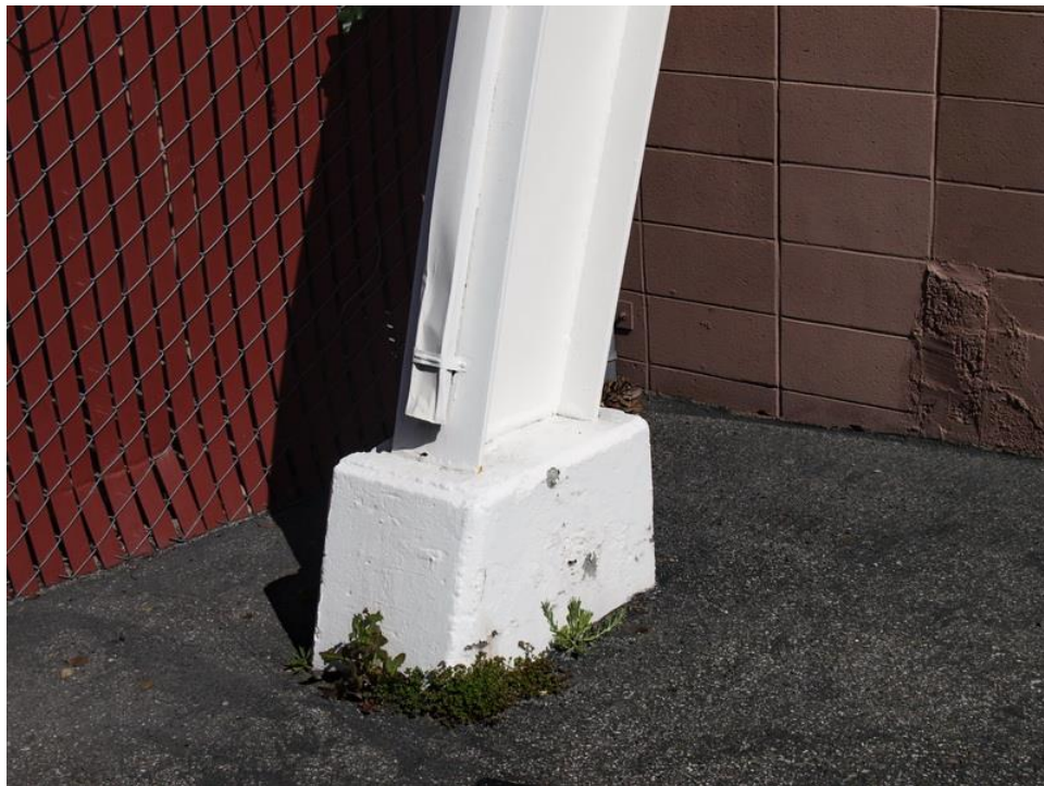
Roof brace detail at ground level.
