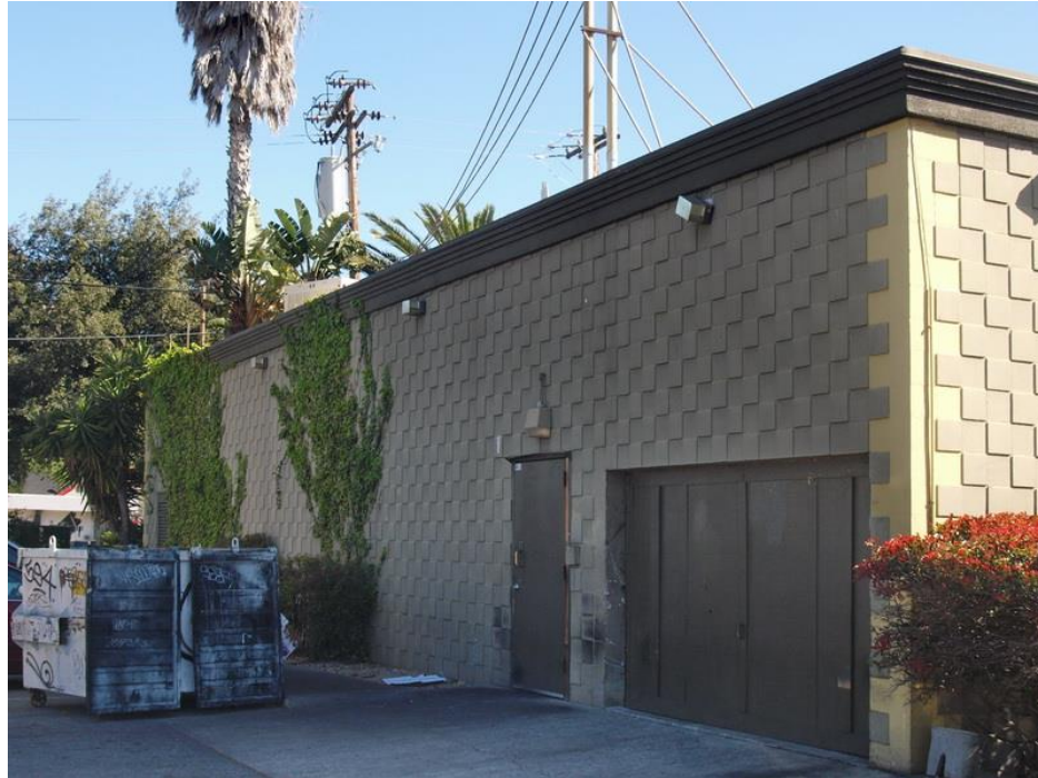
Service entrance at rear of building, viewed facing northeast.
