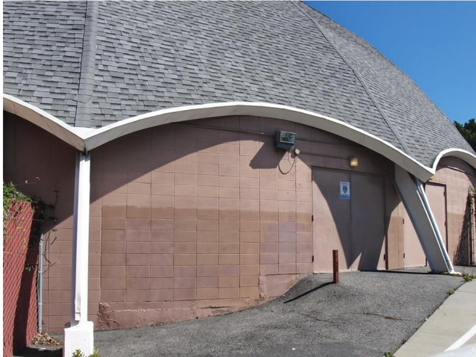
Main dome roof and bracing.
