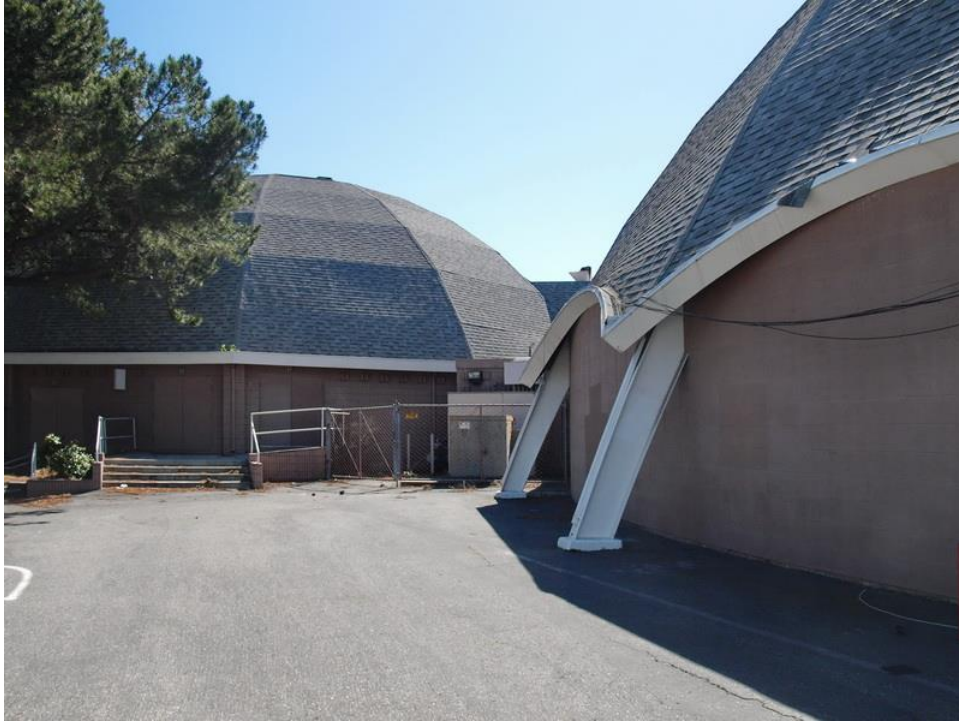
Rear view of north and main domes, viewed facing east.
