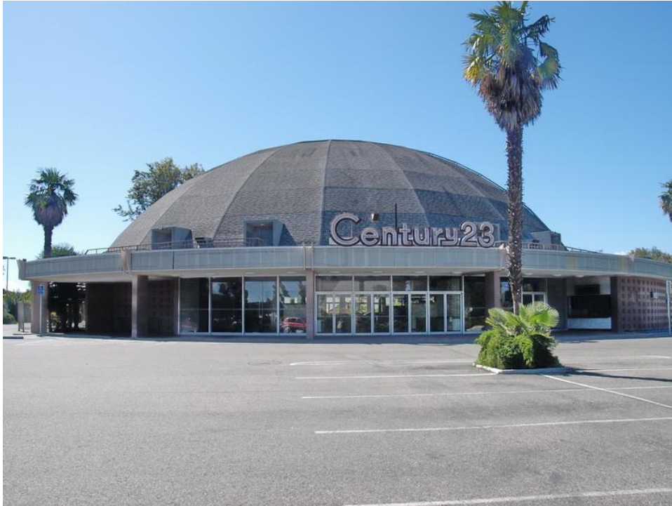
Front elevation, viewed facing south.
