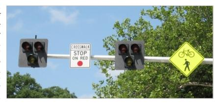
When a pedestrian pushes the button, the HAWK beacon sequence is started, first with flashing yellow followed by steady yellow, then steady red extending for a period of several seconds, and finally by
