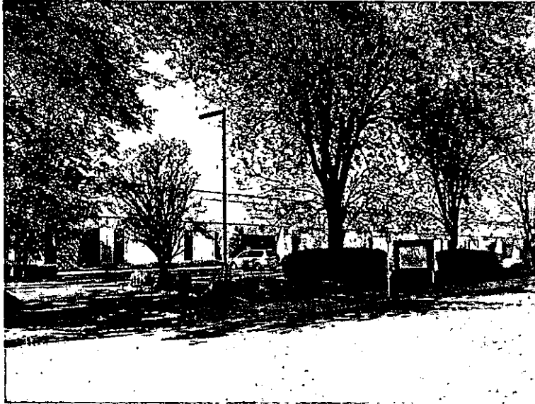
Photograph: APE# 7 Address: 1895 Dobbin Drive APN: 254-55-010 View: Front façade, of the vacant industrial warehouse building. Age: 23 yrs. Constructed in 1984. Camera pointing: NW Date of Photograph: 2/3/07
