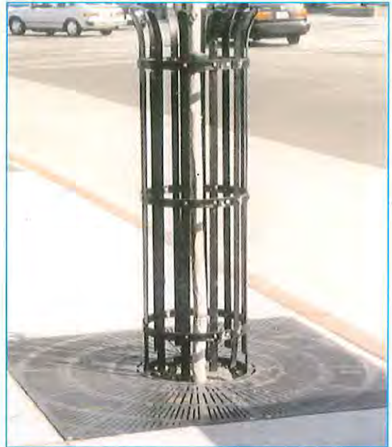
The approved San Jose tree grate, Boulevard Collection Model R8713 with the approved Model "C" tree guard both from Neenah Foundry
