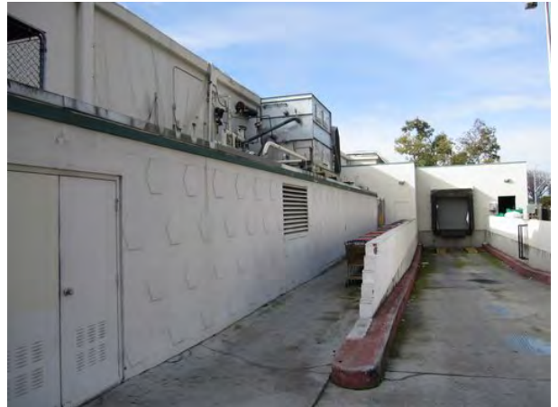
Photograph 6. North side of Safeway showing loading dock.
