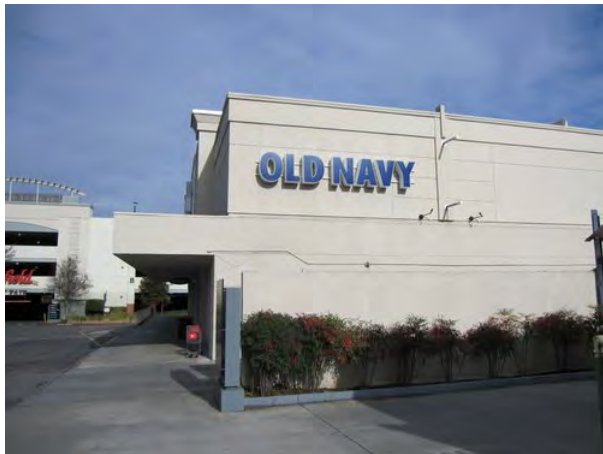
Photograph 13. Old Navy building (looking north).
