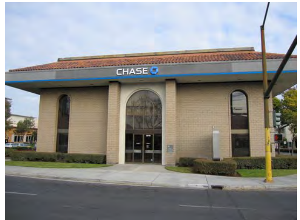
Photograph 2. Chase Bank building (looking north).
