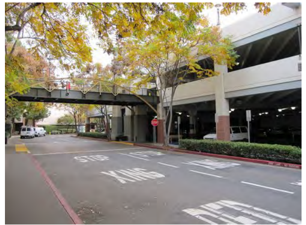
Photograph 4. Parking Structure A (looking east).
