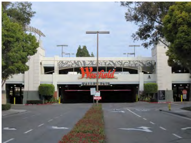
Photograph 3. Parking Structure A (looking north).
