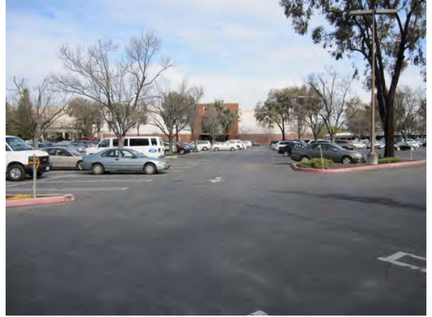
Photograph 18. Parking area on east side of Site (looking northeast). Macy's women's building is shown at center.
