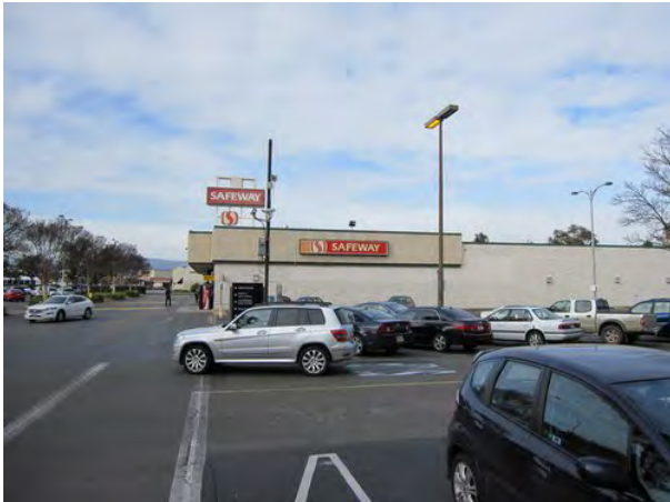
Photograph 5. Safeway and CVS building (looking west).
