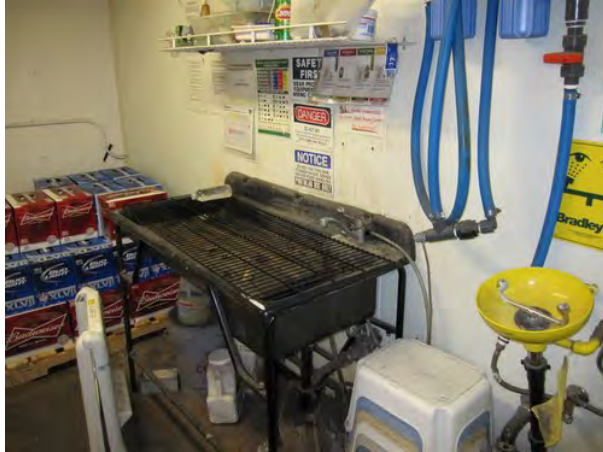
Photograph 11. Photo processing sink in CVS Pharmacy.
