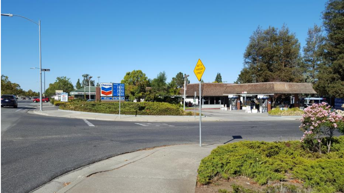
Photograph 1. Existing gas station and carwash on the project site as viewed from the southeast corner of S. De Anza Boulevard and Via Vico
