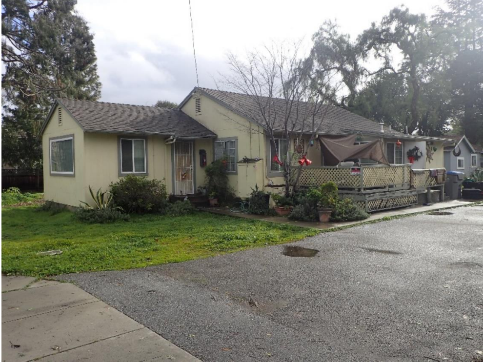
Overview of front house, viewed facing southeast.
