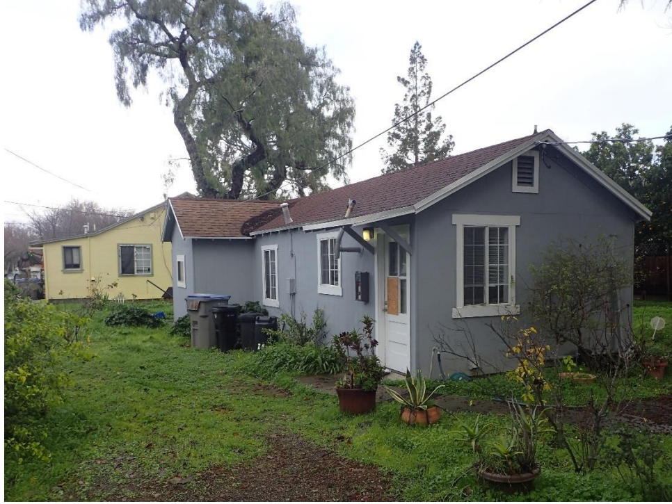
West elevation of second house, viewed facing north.
