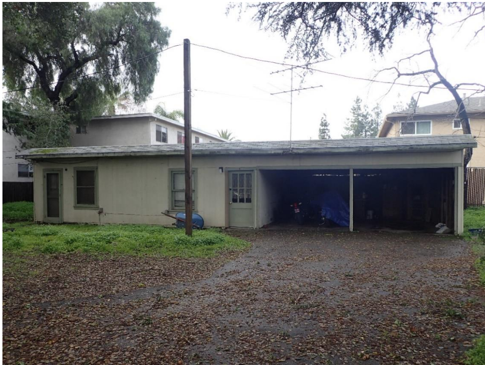
House and carport at southwest corner of site, viewed facing west.
