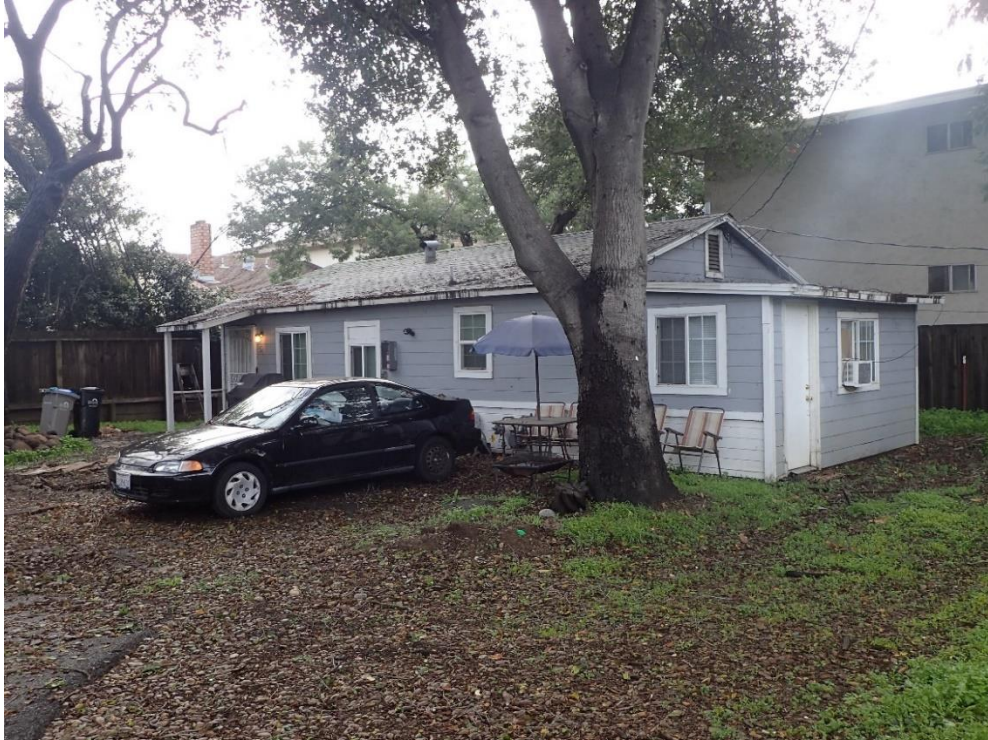
Rear building at southeast corner of site, viewed facing southeast.
