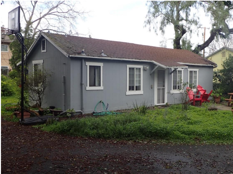
Rear (east) elevation of second house, viewed facing northwest.
