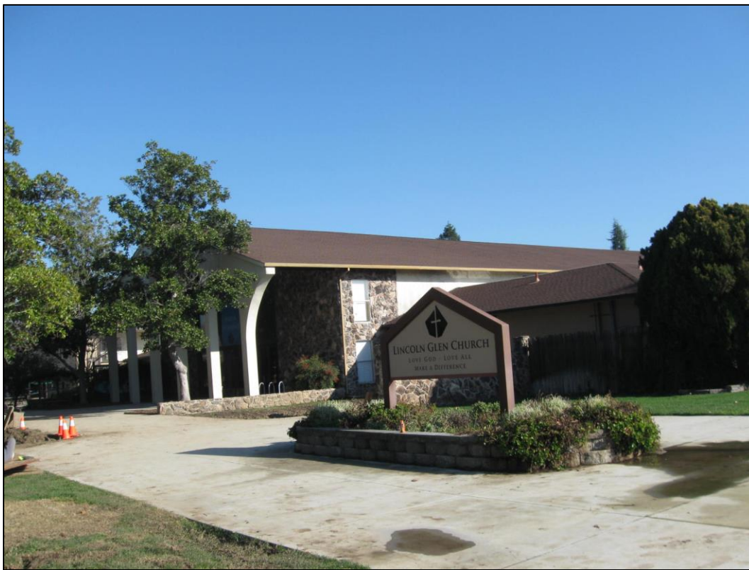
Photograph 6: Adjacent church structure (classrooms, community rooms, offices) to the south of the project site, facing southeast
