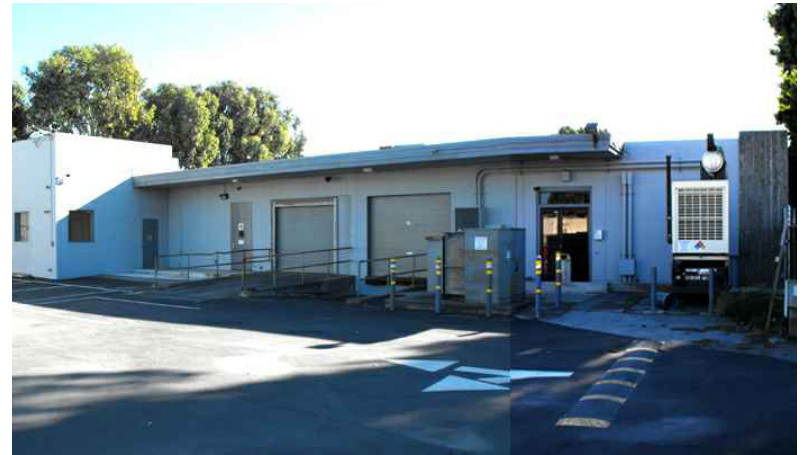
Photo 3: Rear Building Elevation
