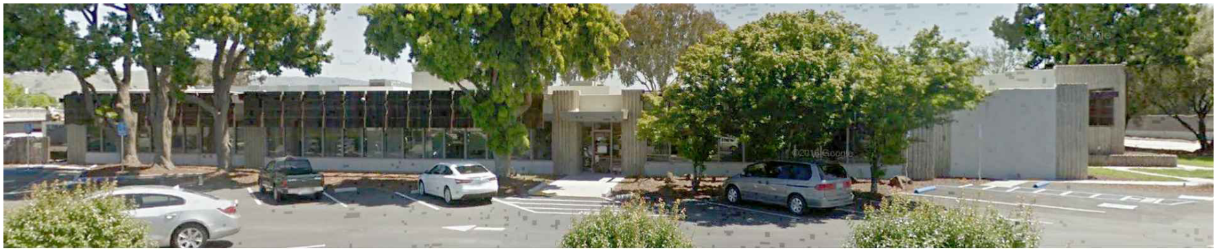
Photo 1: Side Building Elevation
