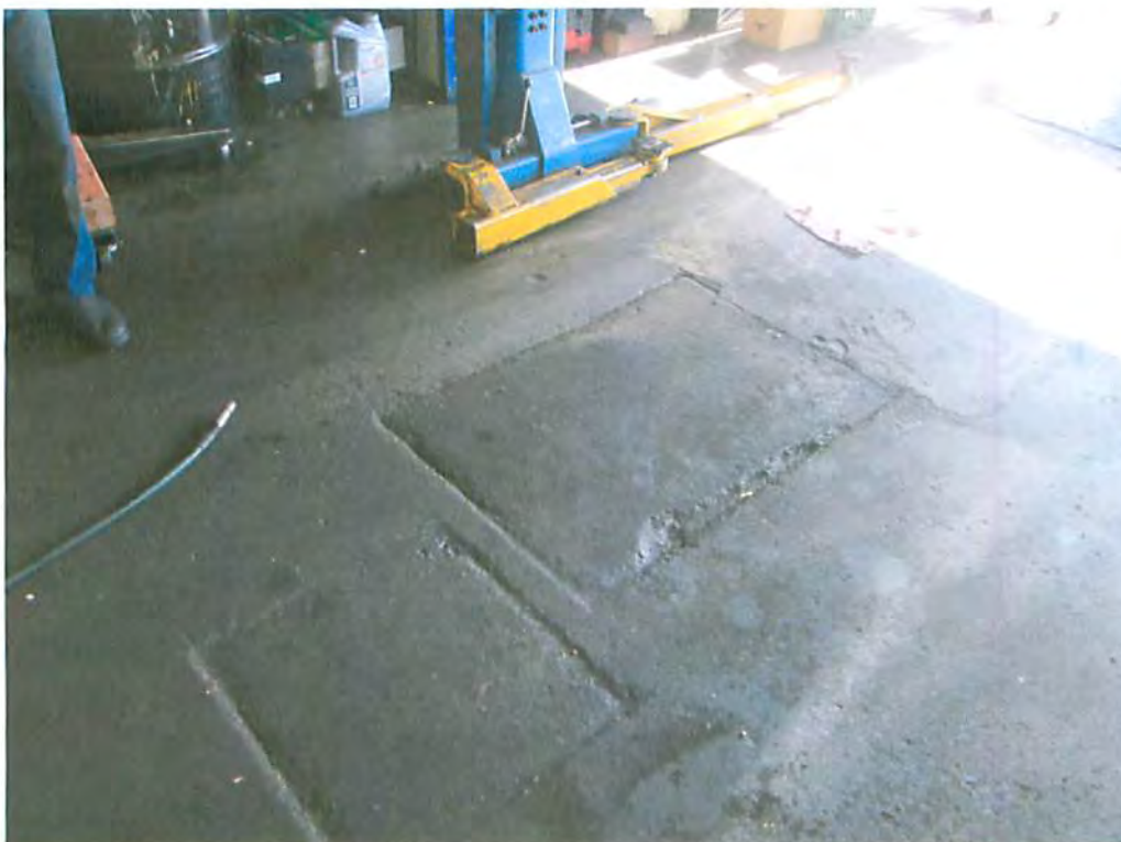
Photo 12: Looking inside the auto repair shop at the concrete floor
