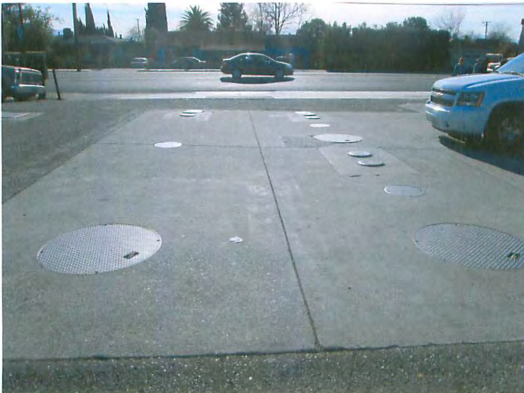
Photo 10: Looking at the underground storage tanks location on the property
