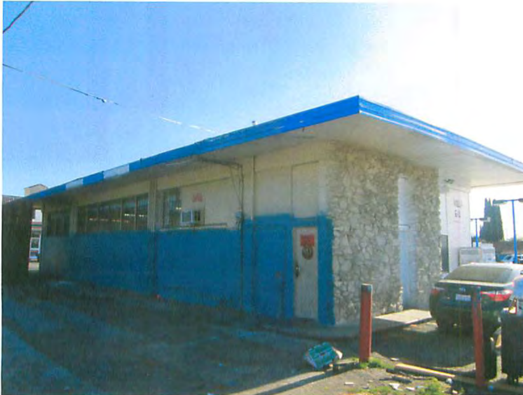
Photo 7: Looking southwest at the behind of the building
