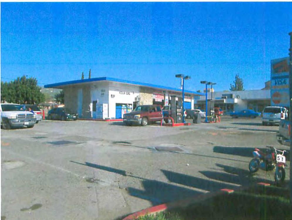
Photo 2: Looking southeast at the Subject Property
