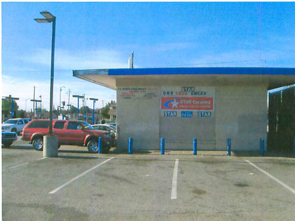
Photo 8: Looking north at the side of the building
