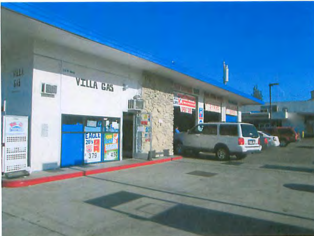
Photo 6: Looking southeast at the Subject Property
