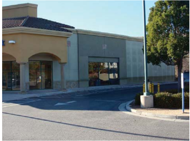
14. View of the northern side of Building 3.
