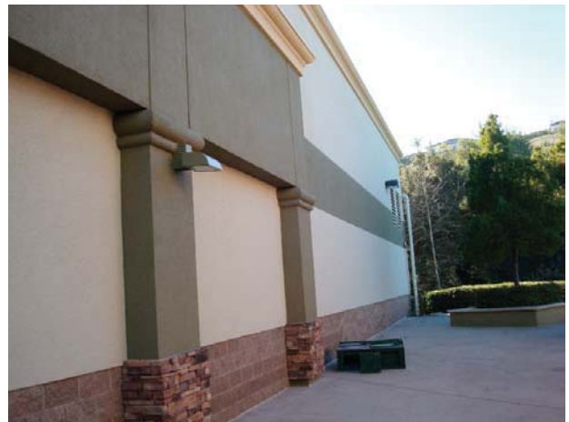
4. View of the western side of Building 1.
