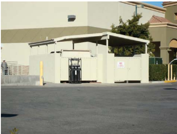
21. View of the garbage compactor enclosure south of Building 1.
