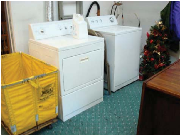
29. Washer and dryer within the dry cleaning facility within Building 2.
