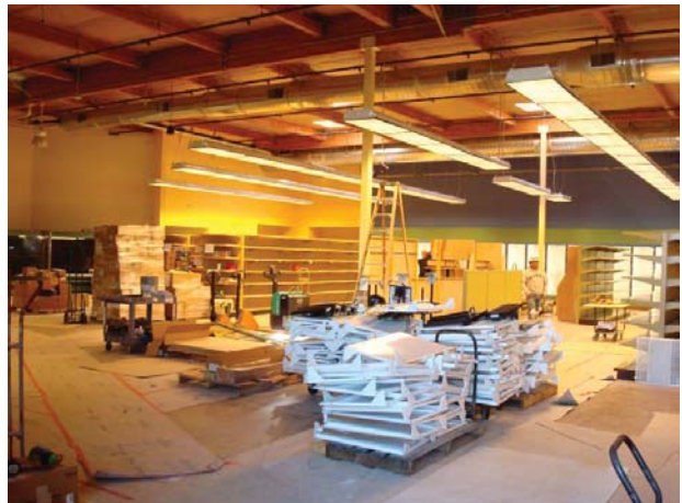
24. Interior of Building 1.
