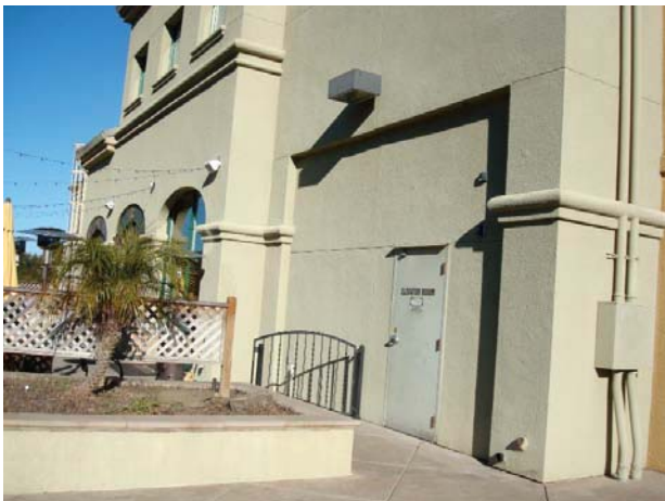
9. View of the southwestern side of Building 2.
