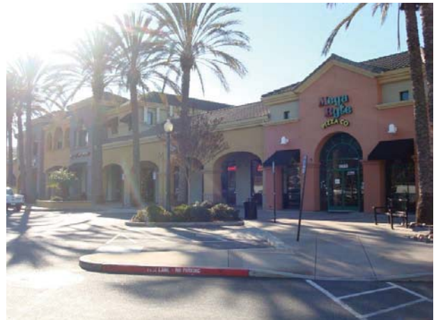
6. View of the northeastern side of Building 2.
