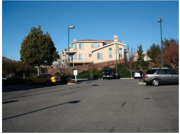
38. View of the adjacent property to the northwest.
