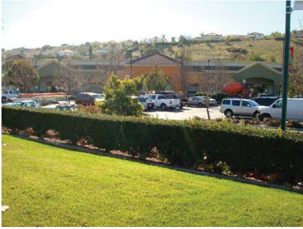
1. View of the northern side of Building 1.
