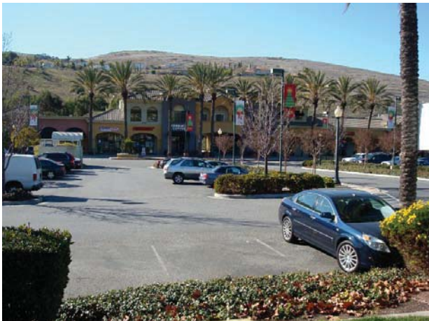
11. View of the northeastern side of Building 2.
