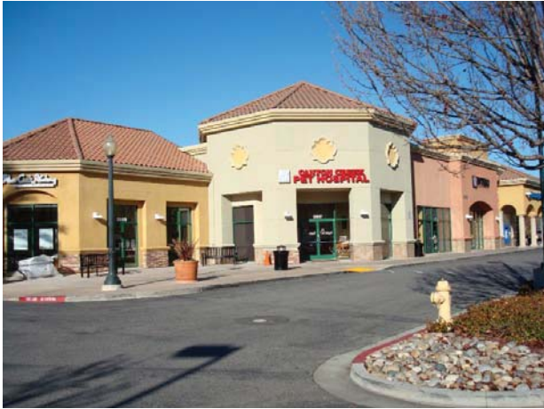
13. View of the eastern side of Building 3.
