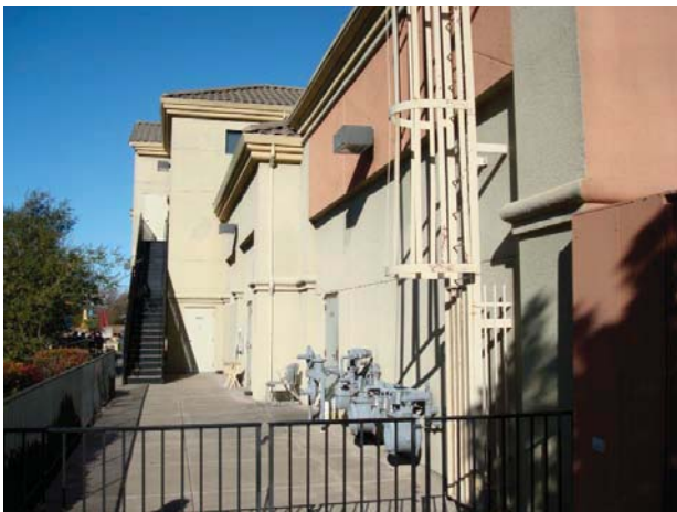
3. View of the southern side of Building 1.
