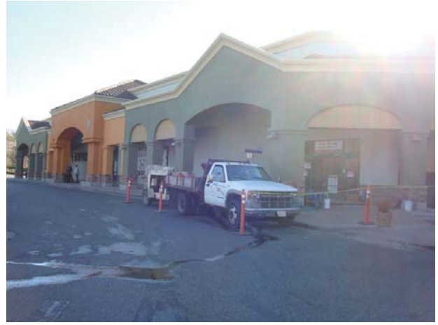
2. View of the northern side of Building 1.
