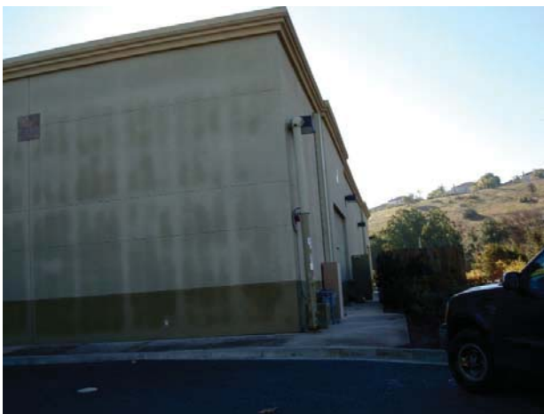
15. View of the western side of Building 3.
