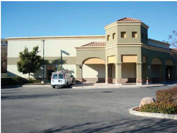
5. View of the southern side of Building 1.
