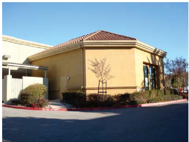
16. View of the southern side of Building 3.
