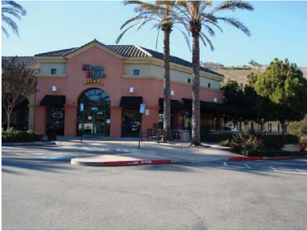
7. View of the northwestern side of Building 2.
