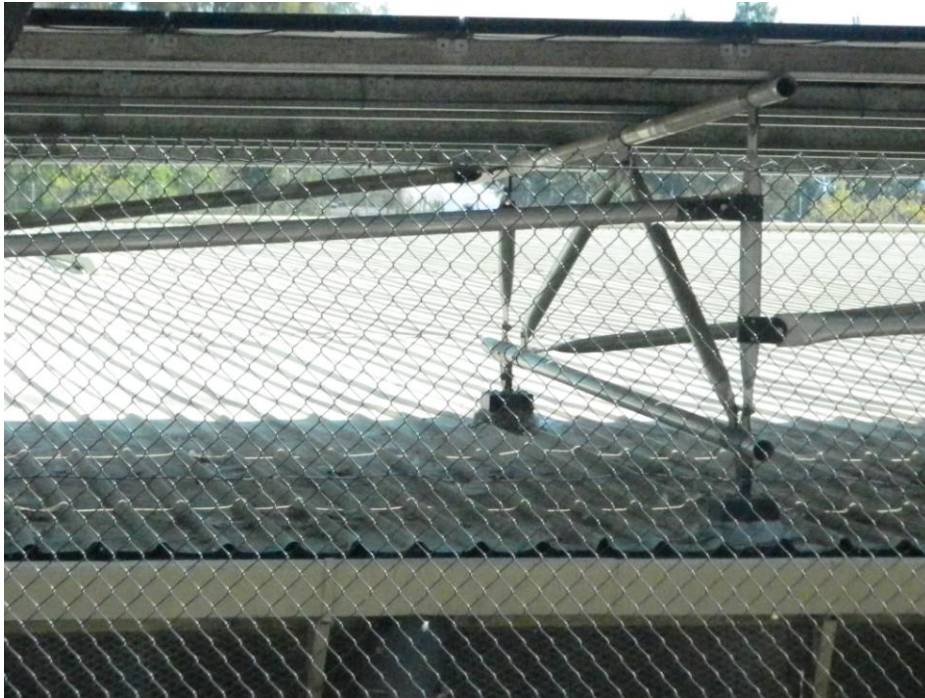
Figure 7 Corrugated metal roof
