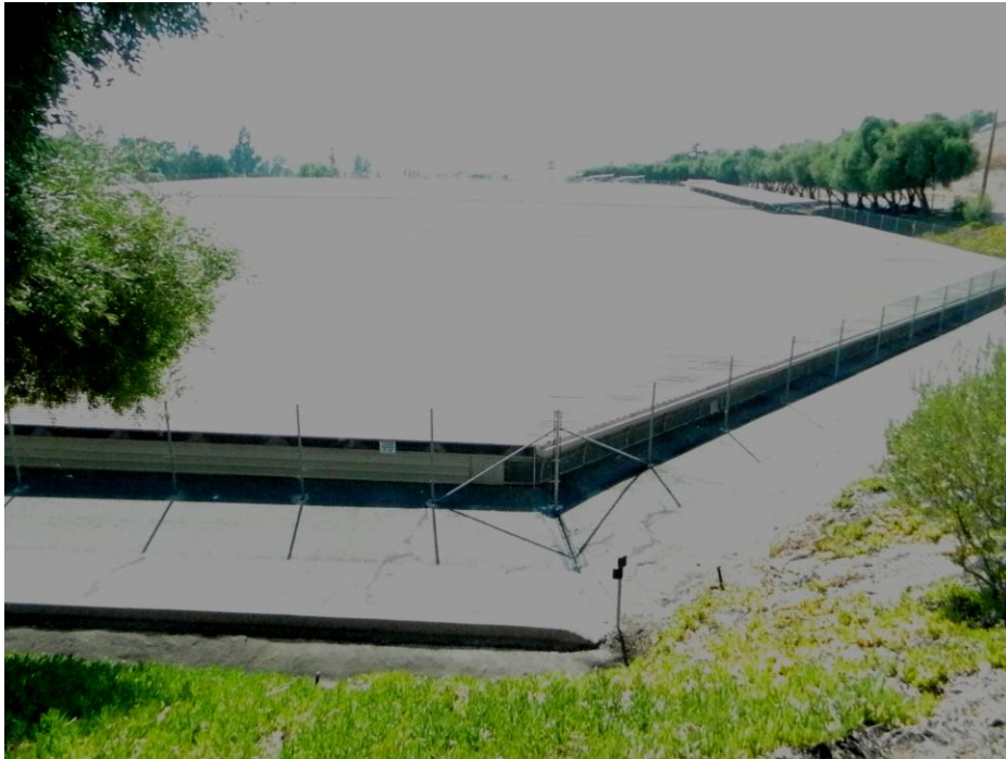
Figure 5 Overview of Columbine Reservoir, facing west (metal roof strongly reflects the sun making photography tricky)
