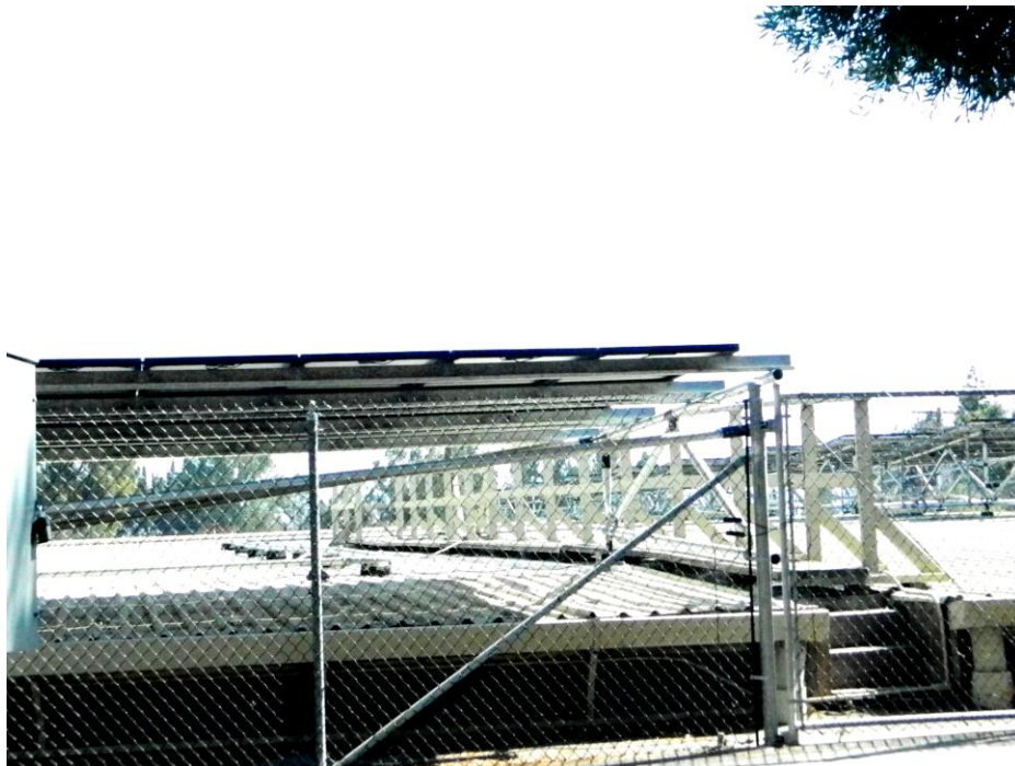
Figure 10 Catwalk along the north section of the roof, facing south
