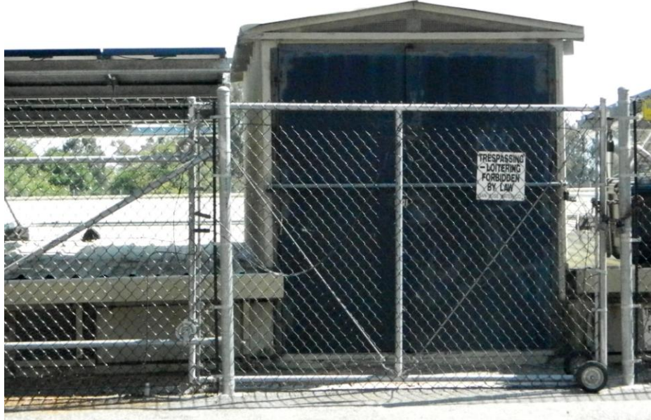
Figure 9 Mechanical building along the north elevation, facing south
