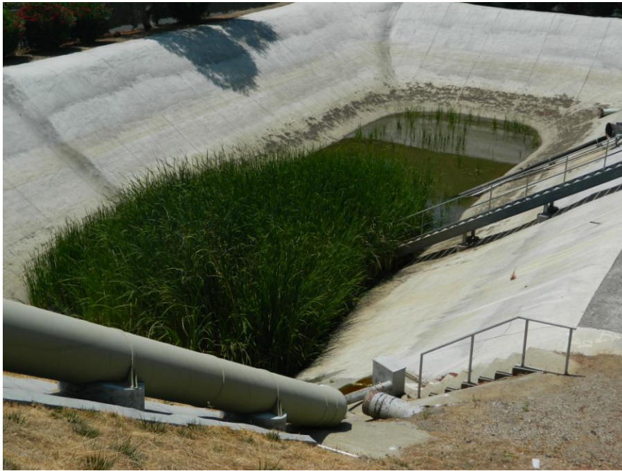
Figure 11. Protected wetland within the earthen and concrete sump within the Project Area
