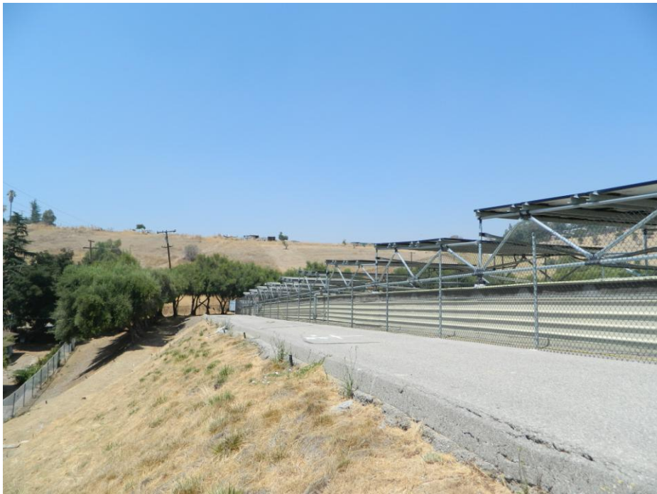
Figure 8 Western Elevation of elevated metal roof and solar modules, facing north
