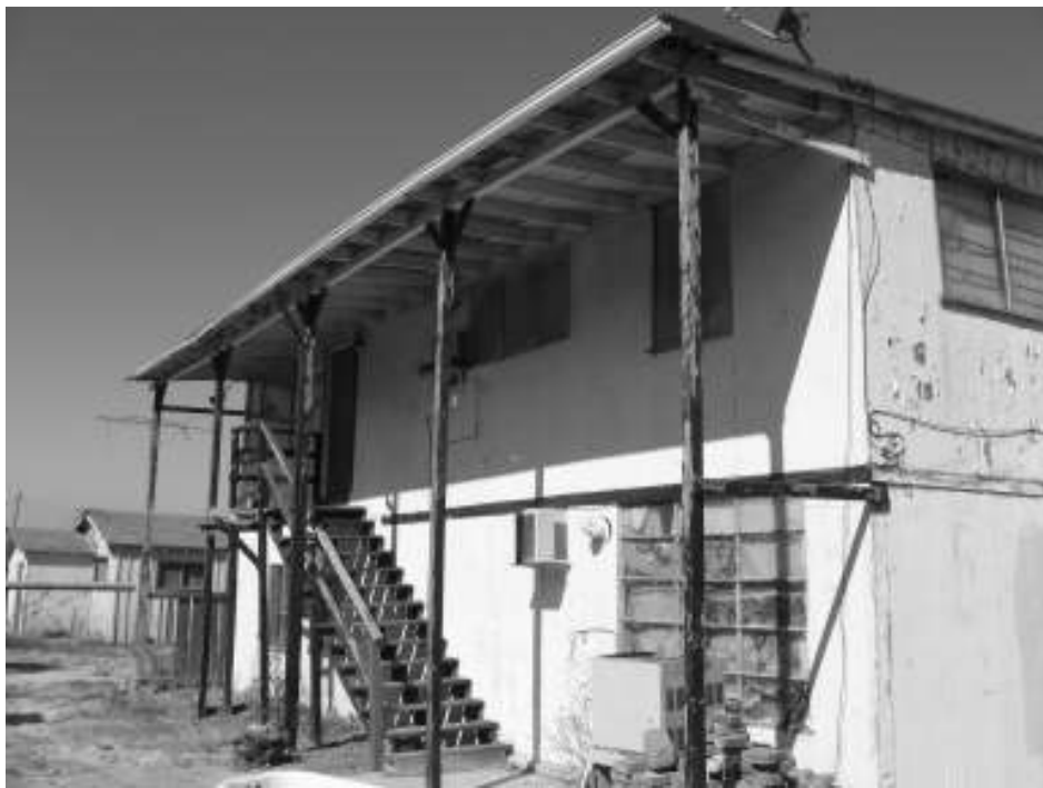
Photo 3: View of the southern addition to the primary residence.
