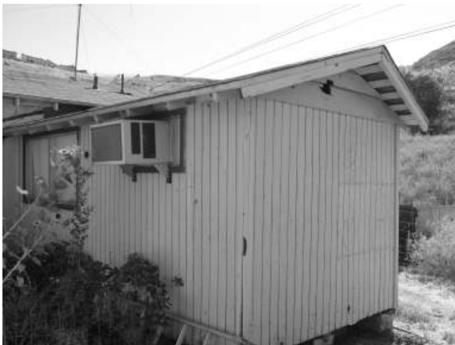
Photo 10: Addition onto the western side of secondary living unit.
