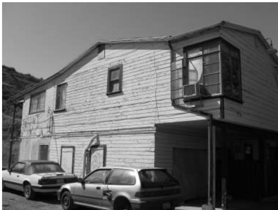
Photo 2: View of the rear façade. Note multi-paned corner window.
