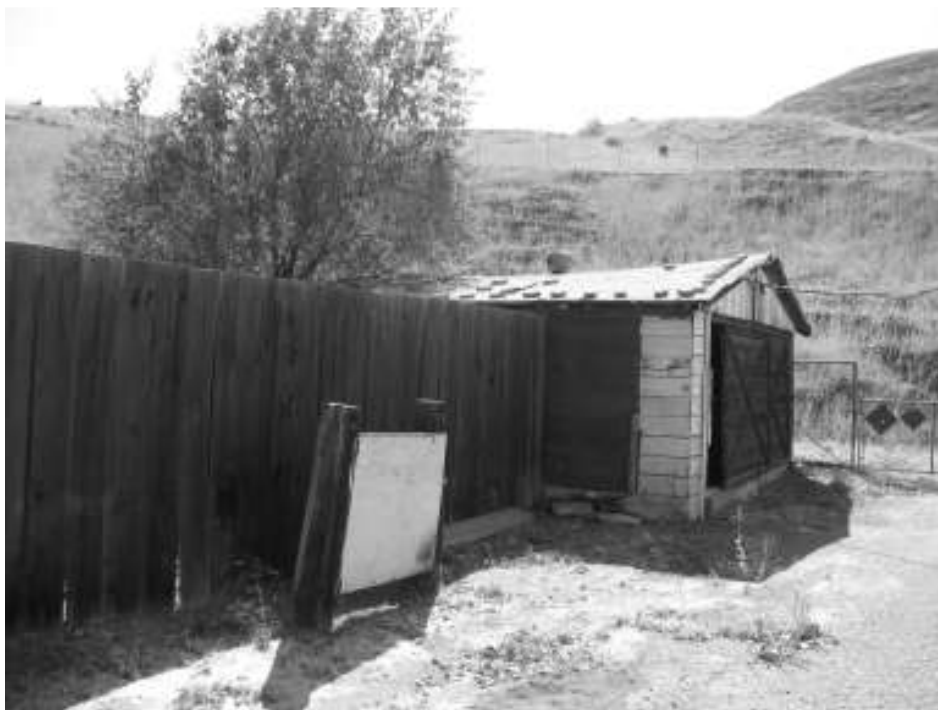
Photo 12: View of large garage/shed behind the main residence.
