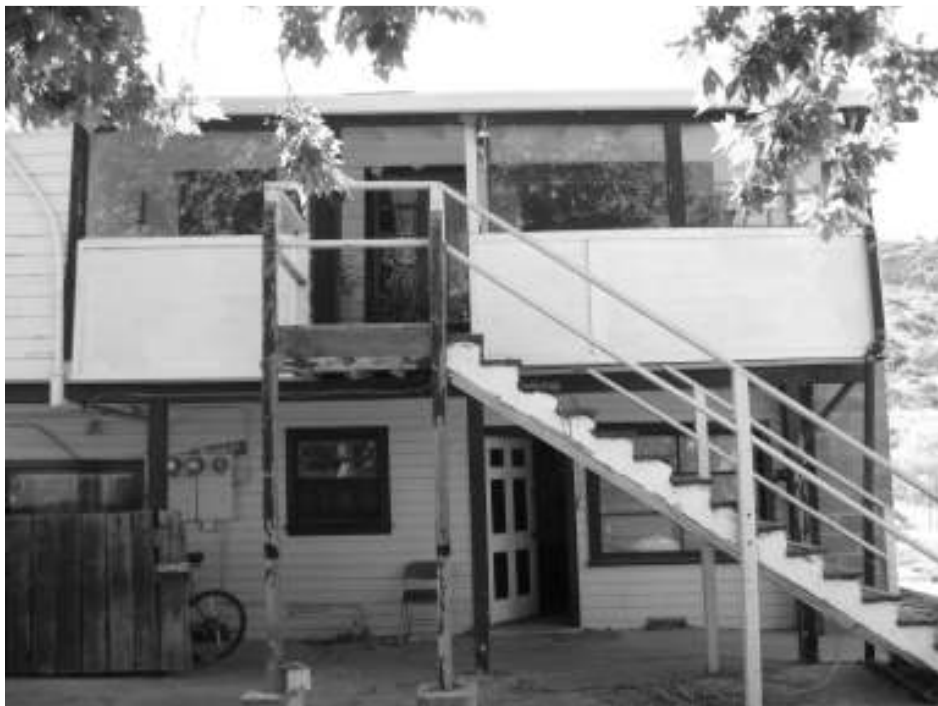
Photo 6: View of the northern façade. Note enclosed upper-story porch.
