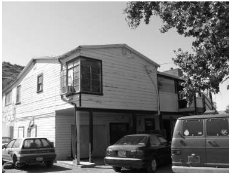
Photo 1: Oblique view of the primary residence from the northeast.
