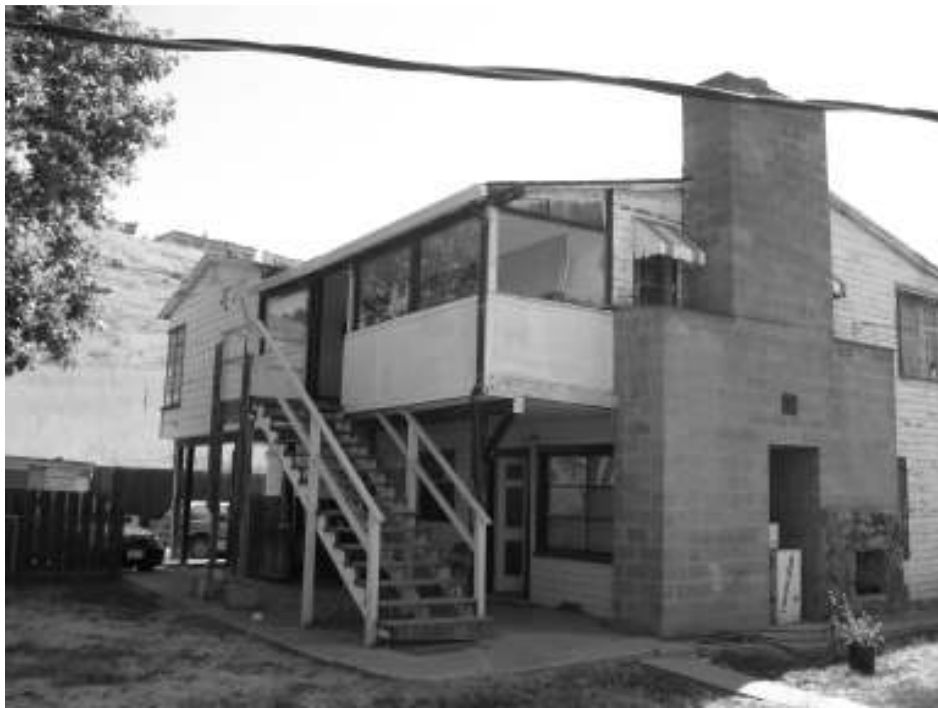
Photo 5: Oblique view from the northwest. Note bifurcated chimney.
