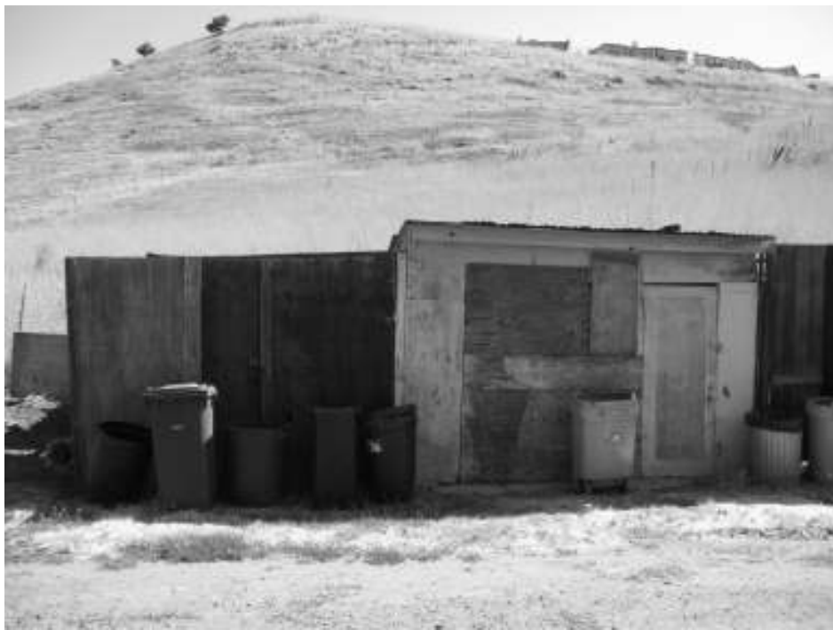
Photo 11: View of the plywood sheds behind the main residence.
